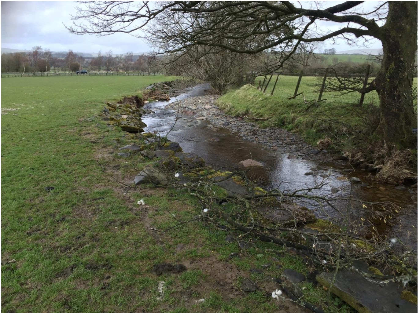
Photograph 7: Raised embankment on the eastern bank of Tebay Gill Beck downstream of the minor road bridge
