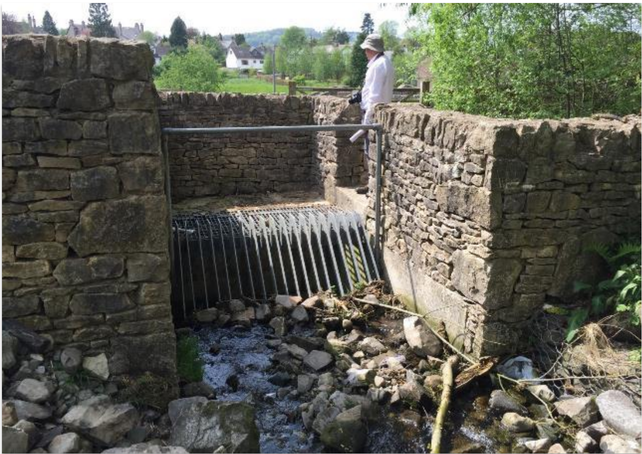
Figure 20: Stock Beck tributary culvert inlet to Stock Beck FSB
