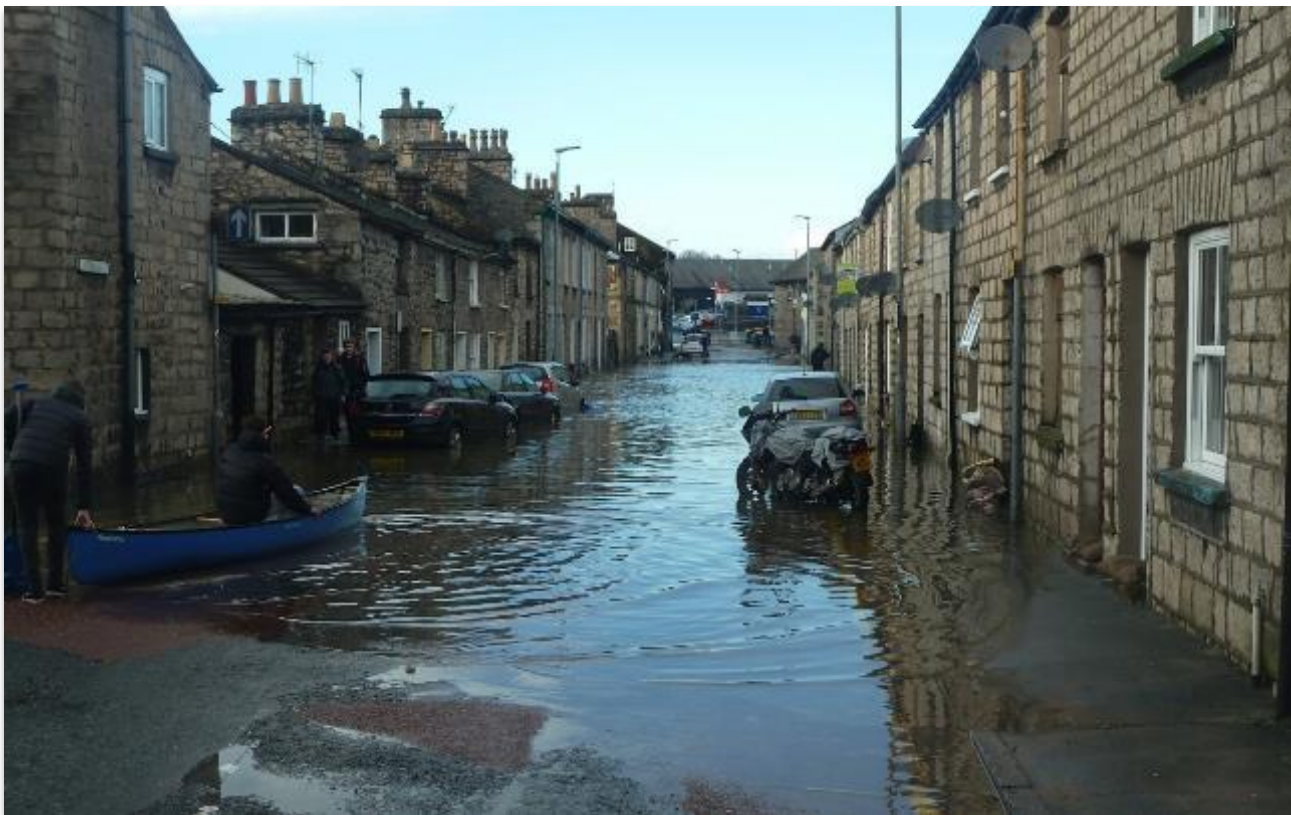
Figure 25: Ann Street in the aftermath of the event on 6 th December 2015
