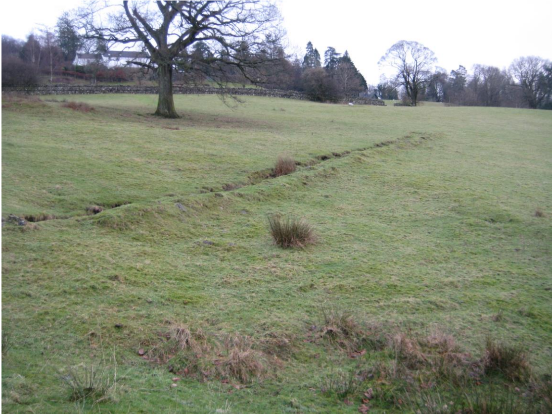
Figure 6 – Flow interception trench on the left bank floodplain of Bell Beck
