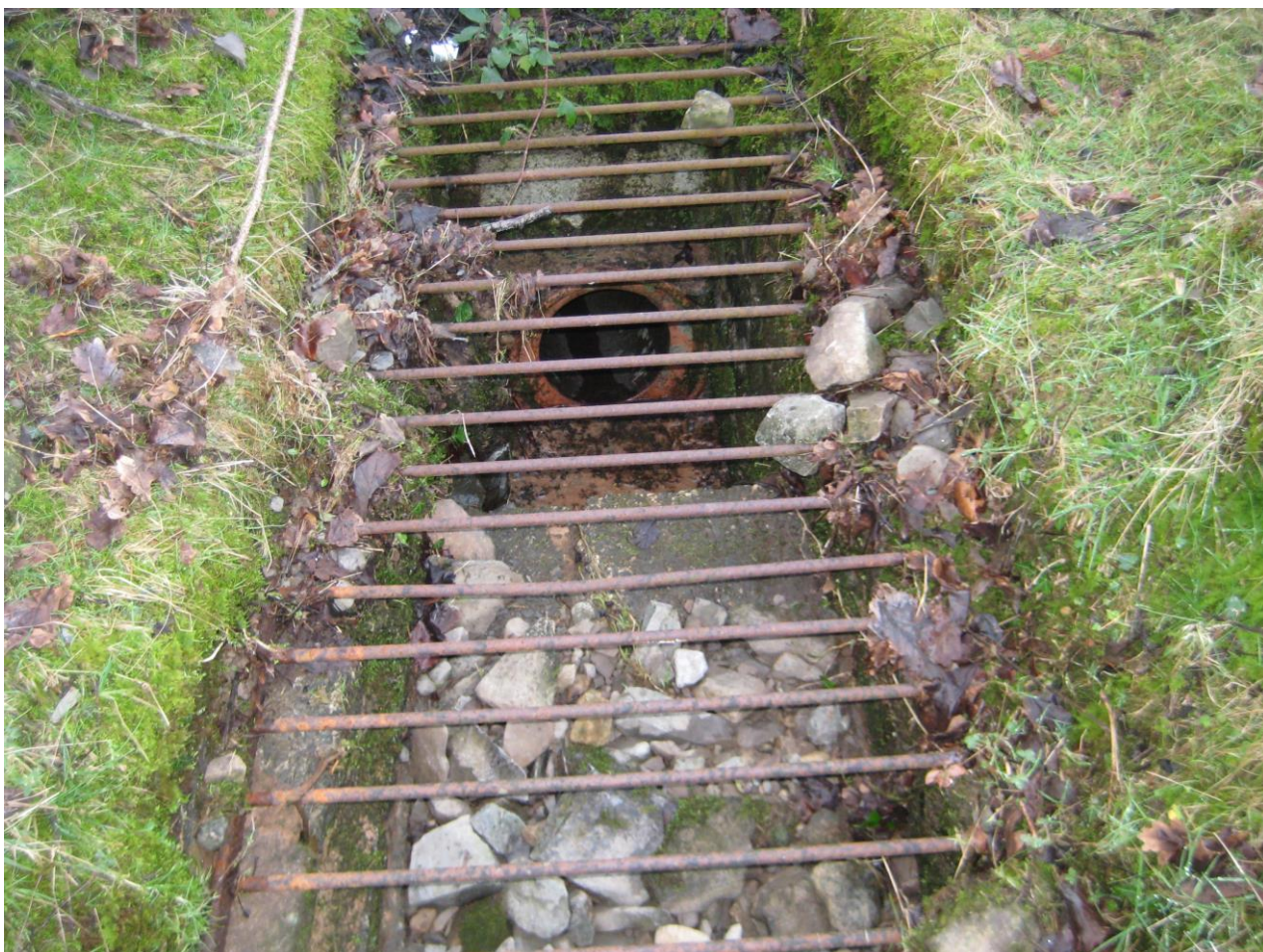
Figure 12 – Culvert inlet and trash screen upstream of the Sun Inn
