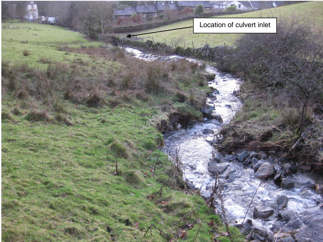
Figure 10 - Bell Beck, looking downstream towards Brook Street (17 th December)
