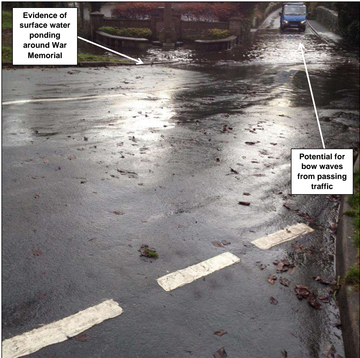
Figure 4: Evidence of surface water flooding around the Beetham War Memorial. Photo taken on 7 th December at 10:36am.
