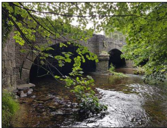
Figure 10: Looking upstream at Beetham Bridge
