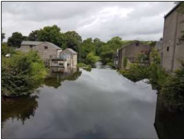
Figure 15: Looking downstream at the Mill Weir
