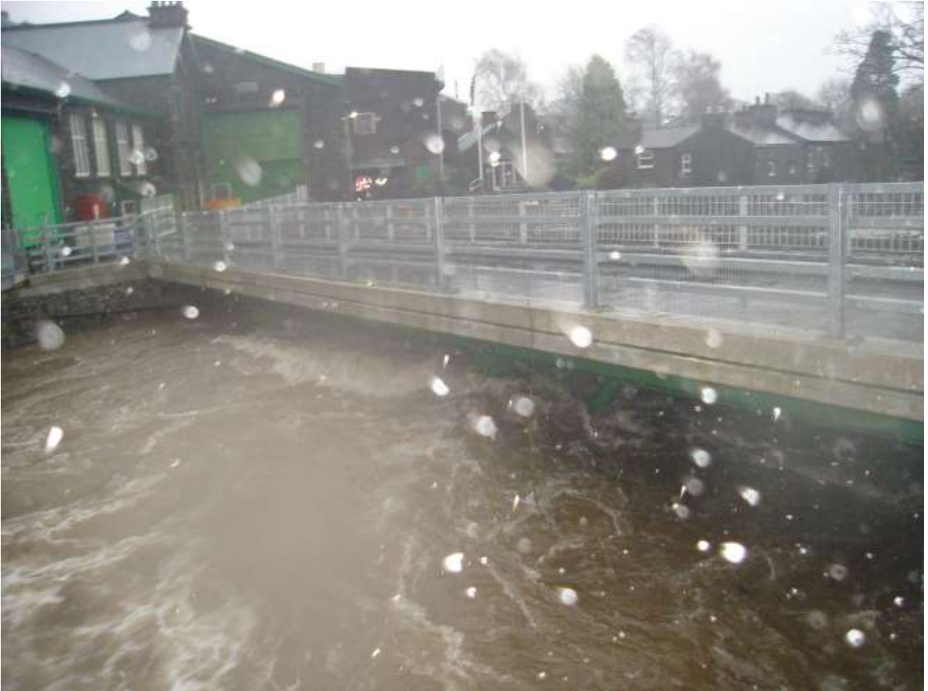
Figure 11: Burneside Bridge at 14:27 on 5 th December
