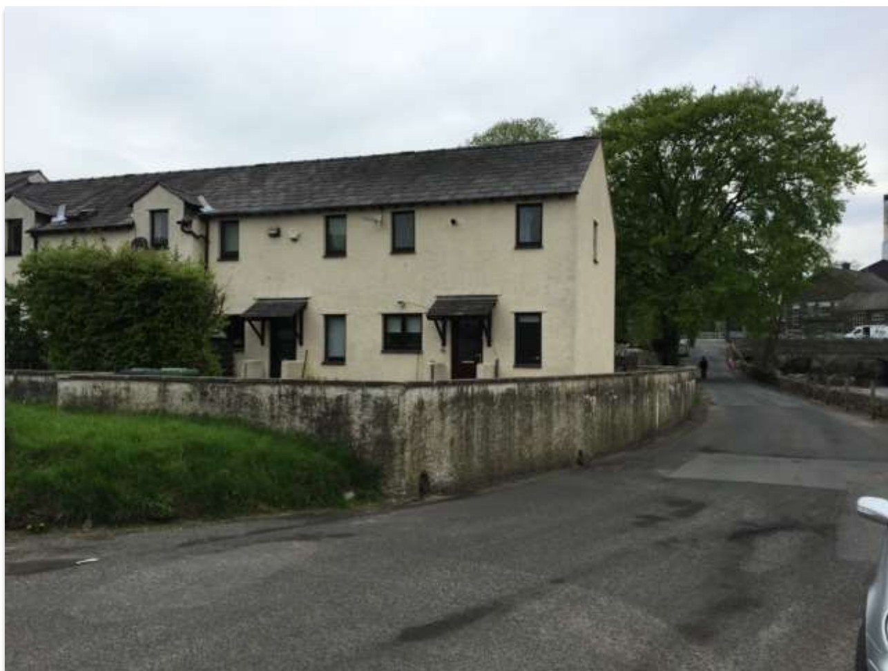
Figure 14: Steeles Row, Burneside, showing existing flood defence wall around properties
