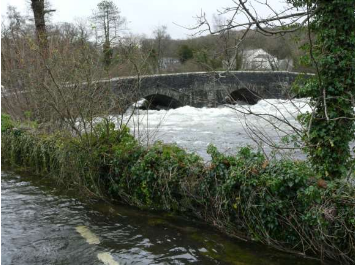
Photograph 12: Newby Bridge, looking upstream from the right bank (Photo courtesy of Zan Fell)
