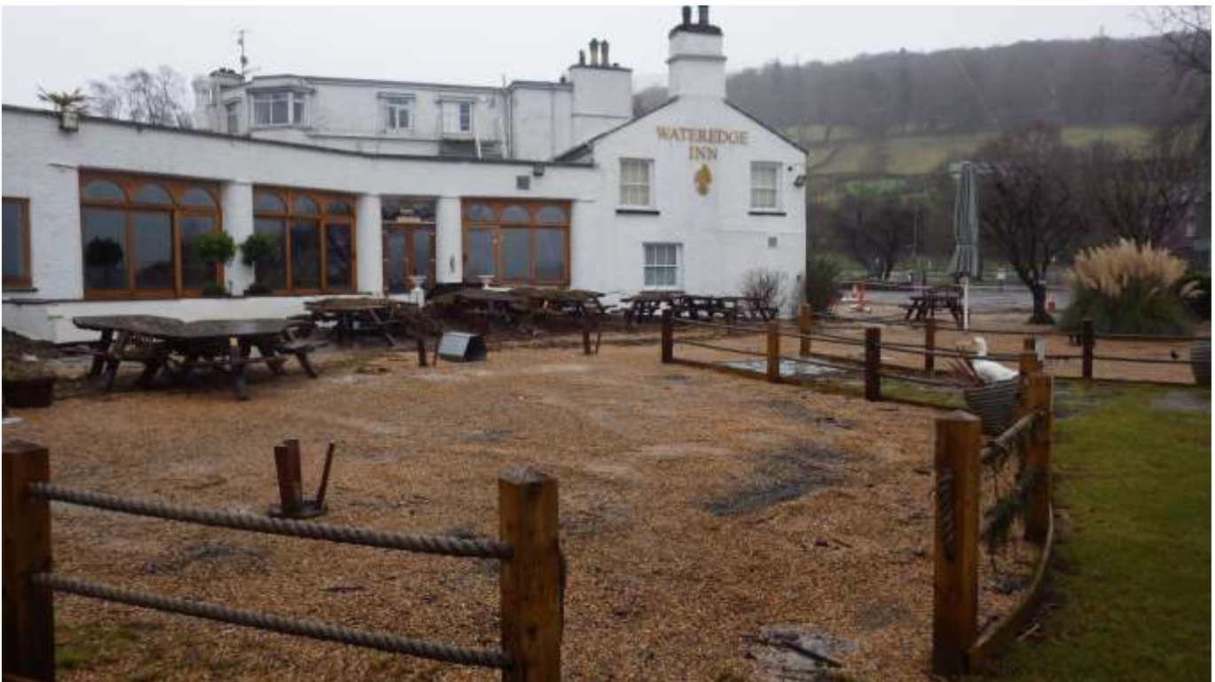
Photograph 1: Debris near the Wateredge Inn shortly after flooding
