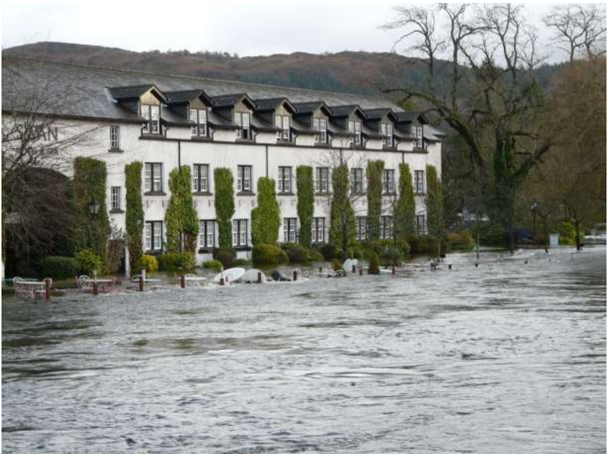
Photograph 16: The Swan Hotel, Newby Bridge
