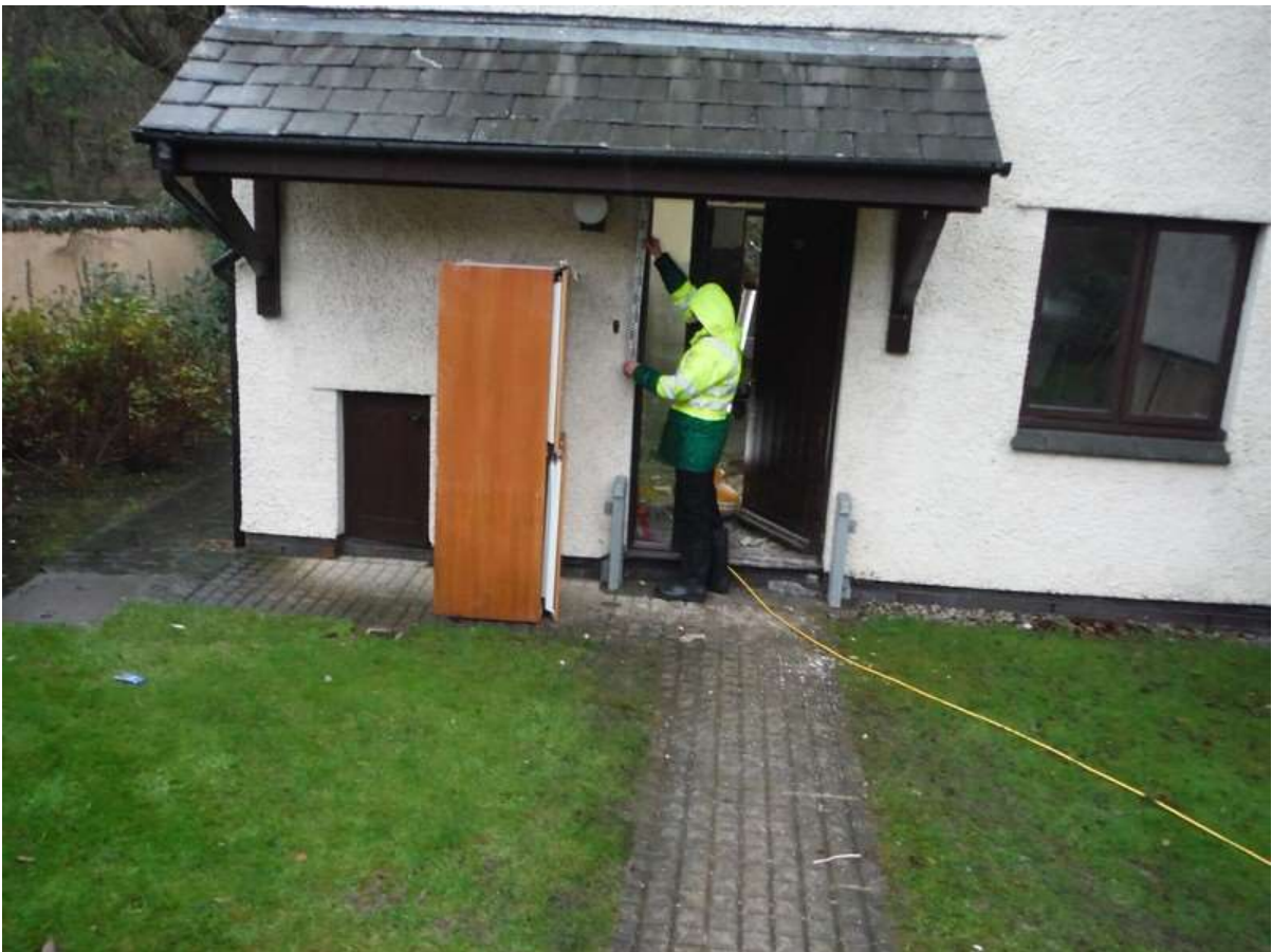
Photograph 21: Backbarrow – Lakeland Village timeshare estate with water mark
