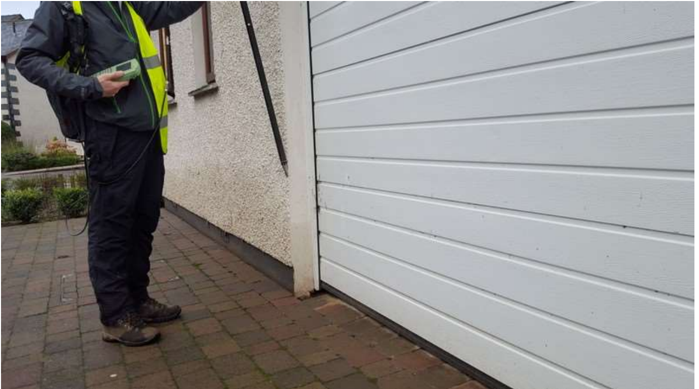
Photograph 8: Flood level on one of the buildings in The Marina
