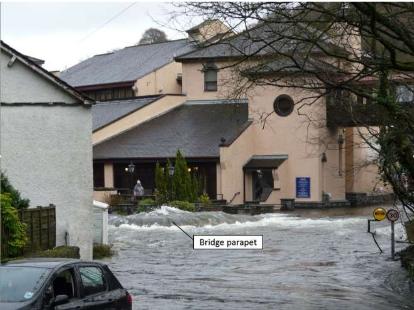
Photograph 18: Backbarrow Bridge – Water overtopping the bridge parapets (Photo courtesy of Zan Fell)
