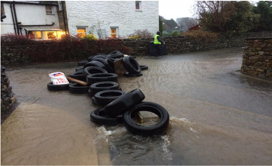
Image 7 – Temporary barrier to protect properties on Guldrey Lane
