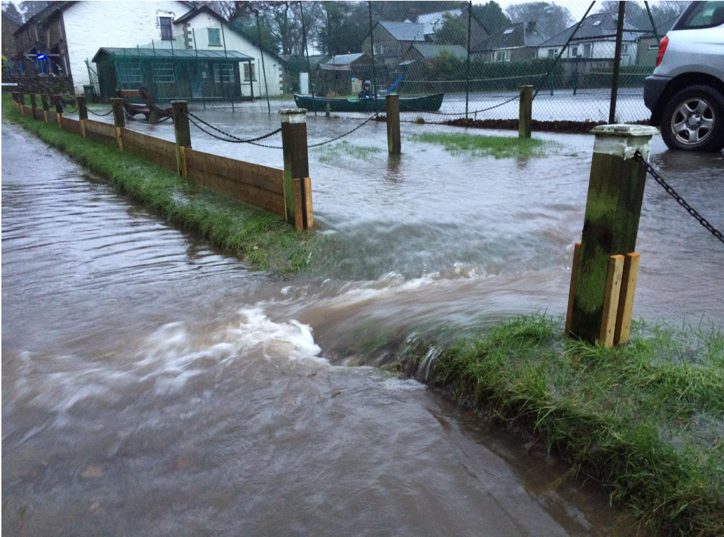
Image 5 – Shows the location where the watercourse exceedance from The Nook joins the overland flows from the footpath.
