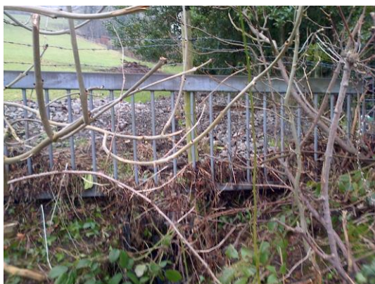
Image 1: Shows the amount of debris trapped on debris screens upstream of Howgill Road
