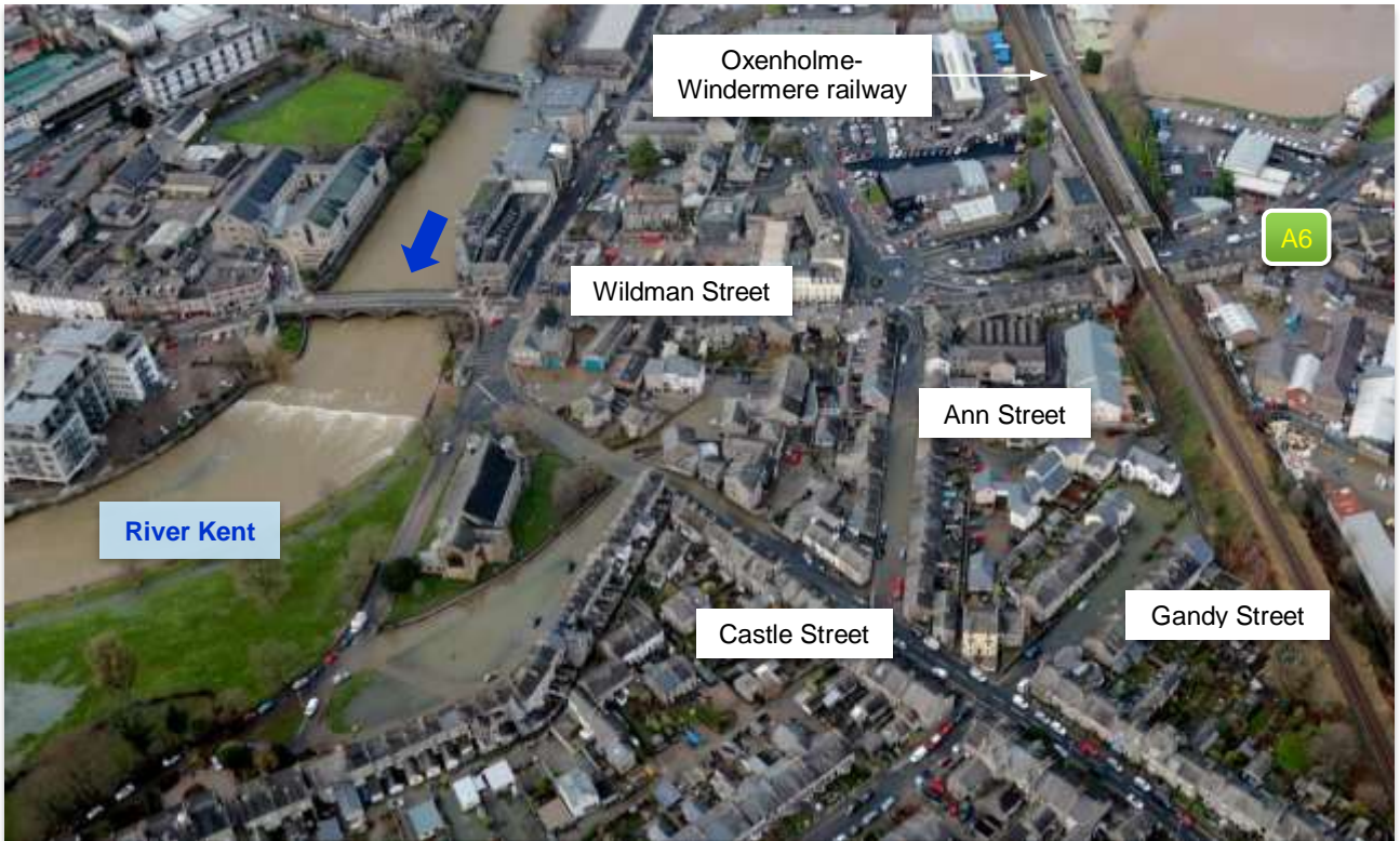
Figure 24: Aerial photograph of the Ann Street and Castle Street area on 6 th December 2015
