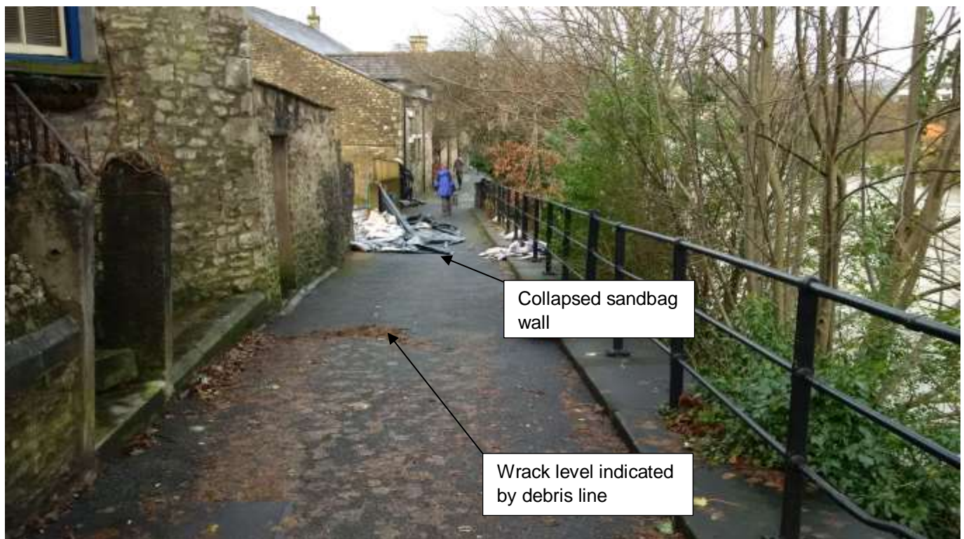
Figure 26: Wrack level on the riverside path at Benson Green, adjacent to Victoria Bridge. Note the sandbag wall which has collapsed towards the river.
