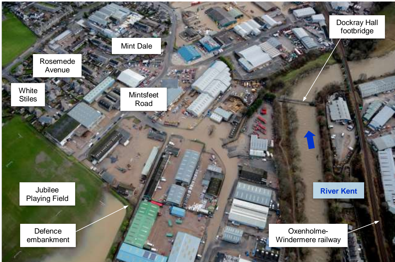
Figure 13: Aerial photograph from 6 th December showing the flooding in Mintsfeet and the existing flood defence embankment along the south and western boundaries of the Jubilee Playing Fields
