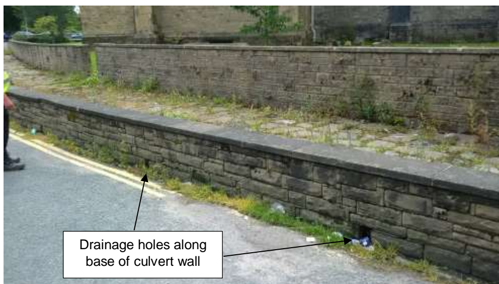
Figure 23: Redundant Stock Beck culvert on Castle Crescent
