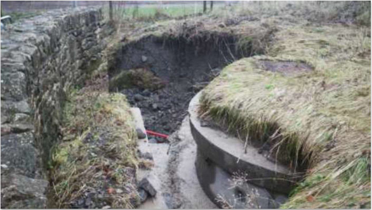
Figure 21: Scour damage to rear of outfall structure upstream of Stock Beck FSB
