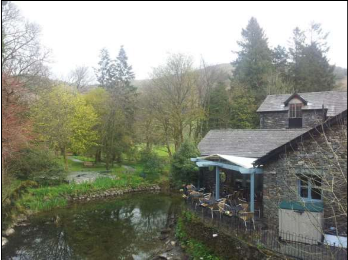
Figure 8 – Looking Upstream from Church Bridge at Riverside Retaining Walls on the River Rothay
