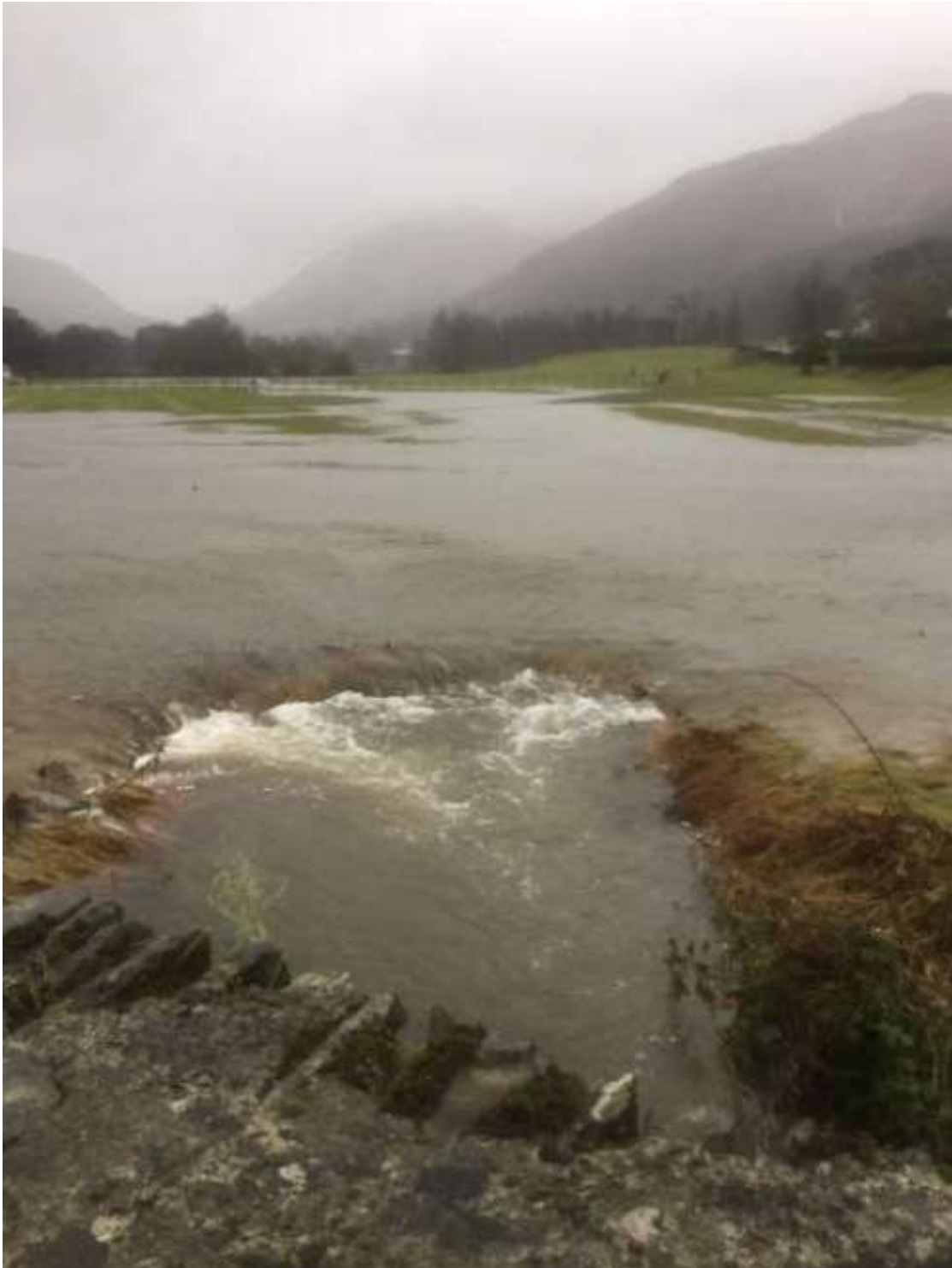
Figure 19 – Overland flow route across the floodplain towards Stock Bridge.
