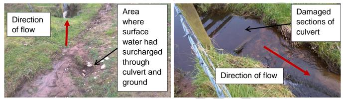
Photographs 11 & 12: Damage at the downstream end of Brown Sike culvert
