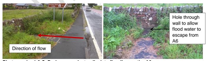
Photographs 4 & 5: Drainage works to alleviate flooding on the A6
