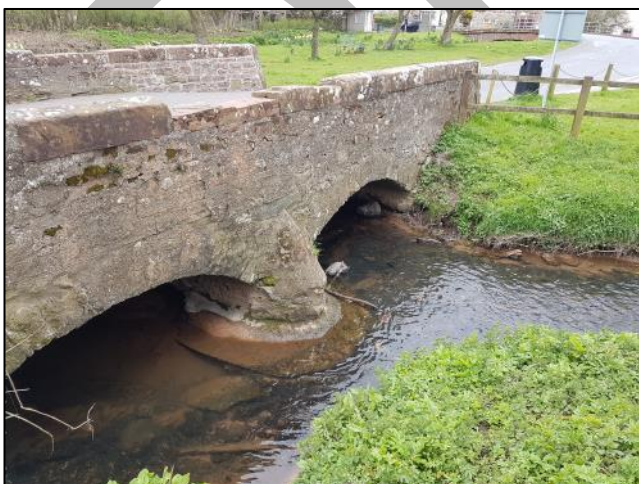
Photograph 9: Warcop Bridge over the Lowgill Beck
