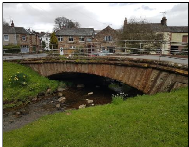
Photograph 10: Bridge over the Crooks Beck looking upstream
