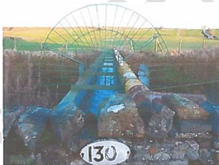
Photograph 1: Aqueduct across railway line
