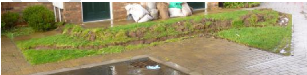
Photograph 5: Evidence of flood diversion works in Birkbeck Gardens
