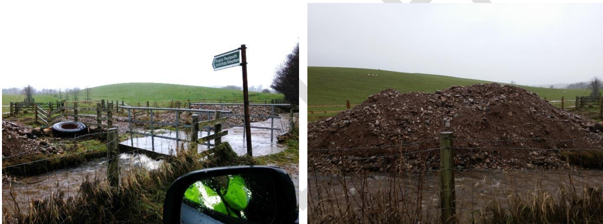
Photographs 10 & 11: Coffin Bridge and gravel that has been removed from Hartley Beck (taken on 10/12/2015).
