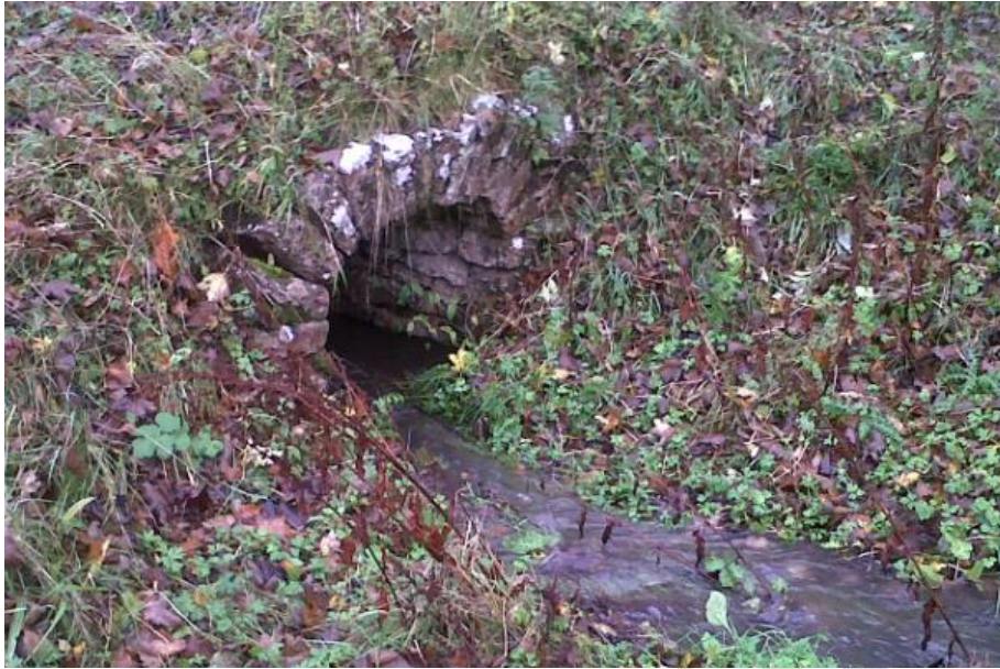
Photograph 1: Culvert entrance upstream of A685
