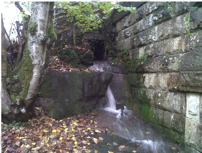
Photograph 2: Culvert discharge at River Eden
