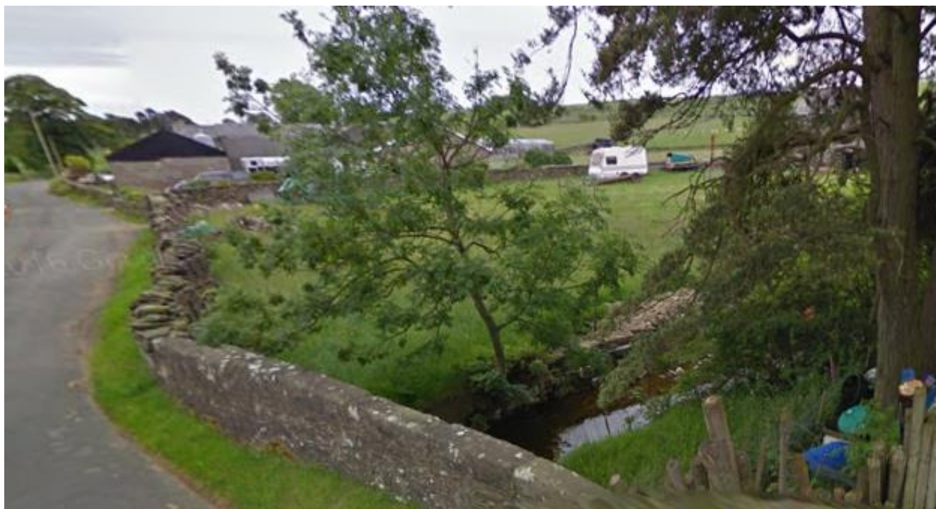
Photograph 11: Minor Road Bridge over Tebay Gill Beck (taken from Google Maps)
