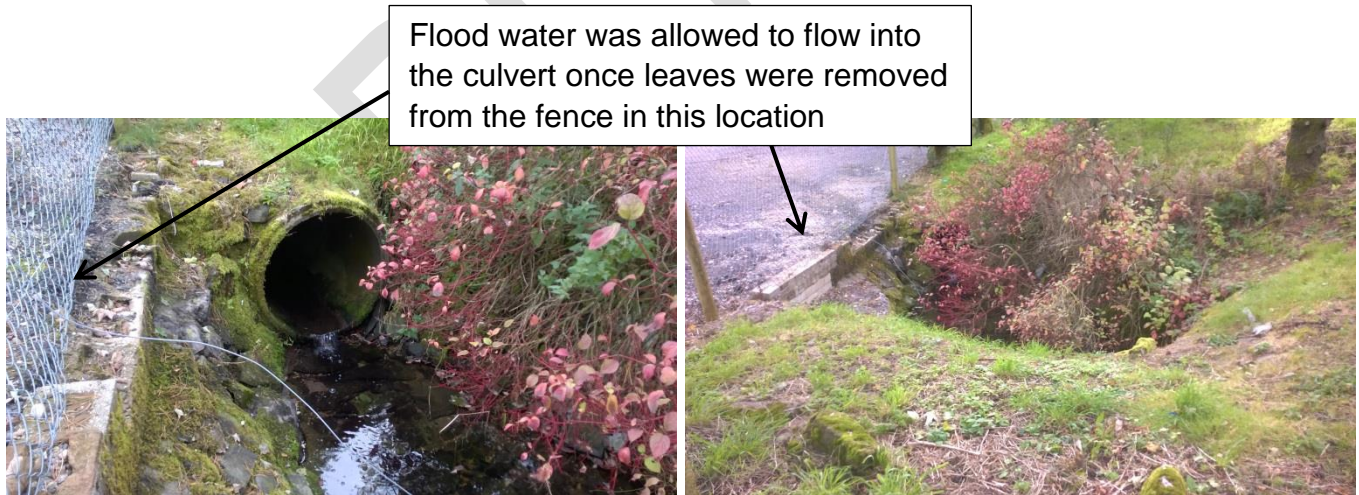
Photographs 6 & 7: Opening between culverts outside the depot, Old Tebay
