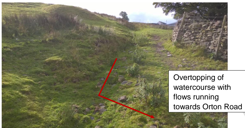
Photograph 4: Watercourse above fell road
