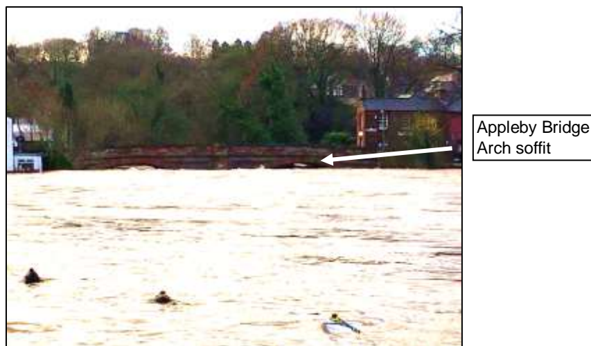
Photograph 12: River level just below the bridge soffit level before the event peak
