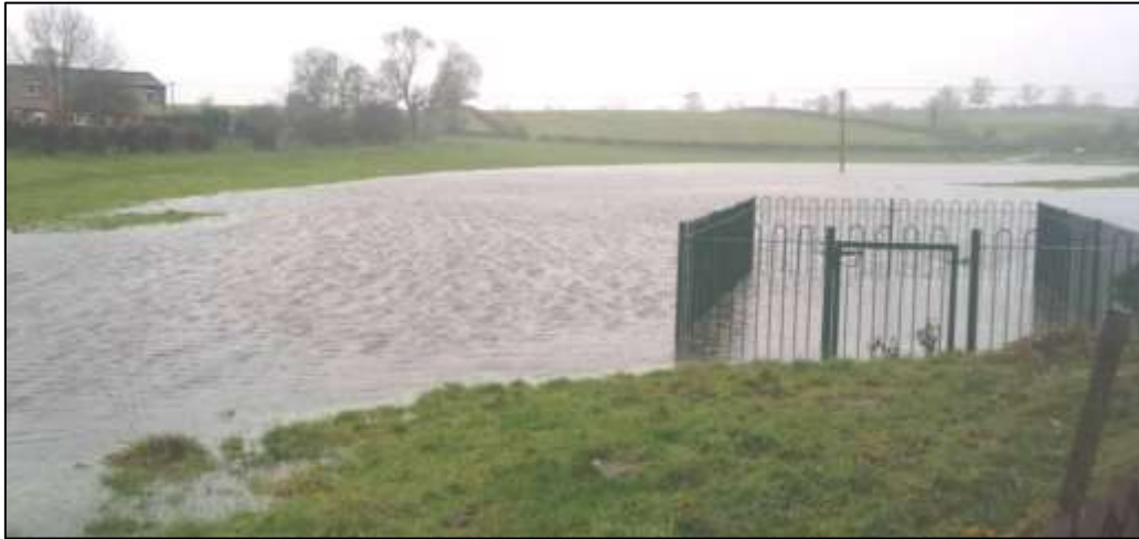
Photograph 10: Doomgate culvert inlet at Colby Lane (2005)
