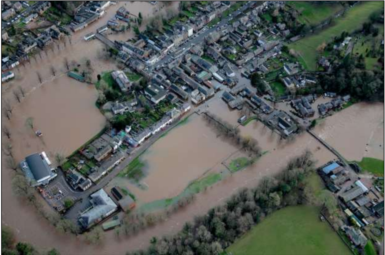
Photograph 30: Flood water from the Eden being held back by the defences. Water ponding behind floodwall on Chapel Street is from Doomgate culvert.
