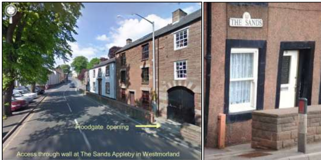
Photographs 1 & 2: Property level flood defence measures introduced. Wall in photo on right is a CCC highways wall not part of DEFRA pilot
