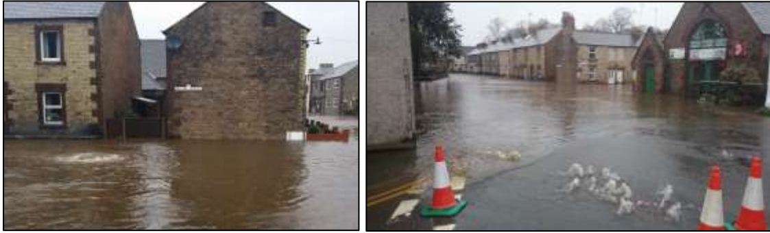
Photographs 5 and 6: Doomgate Culvert Manhole Surcharged, 11:00hrs (left) and 13:30 (right) on 5 th December
