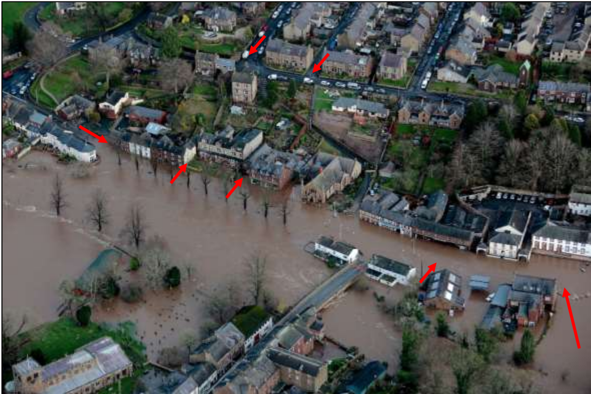
Photograph 4: Flood at the Sands, Appleby
