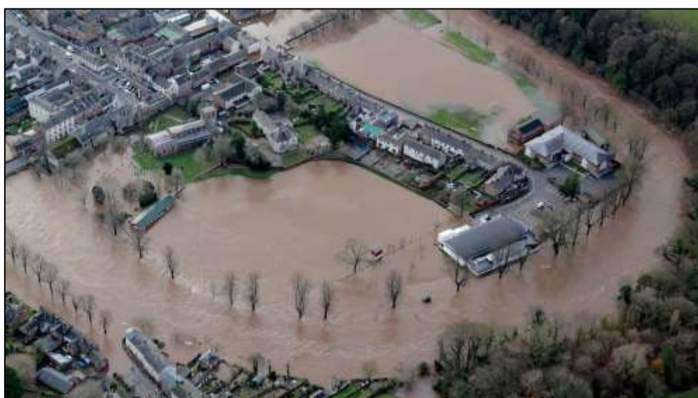
Photograph 28: Flood Extent at Cricket Field
