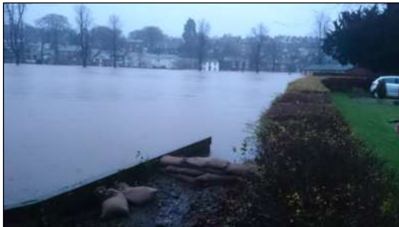
Photograph 18: Embankment Settled at Cricket Ground – 15:44hrs on 5 th December 2015
