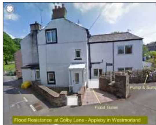
Photograph 11: Properties on Colby Lane - Property level measures
