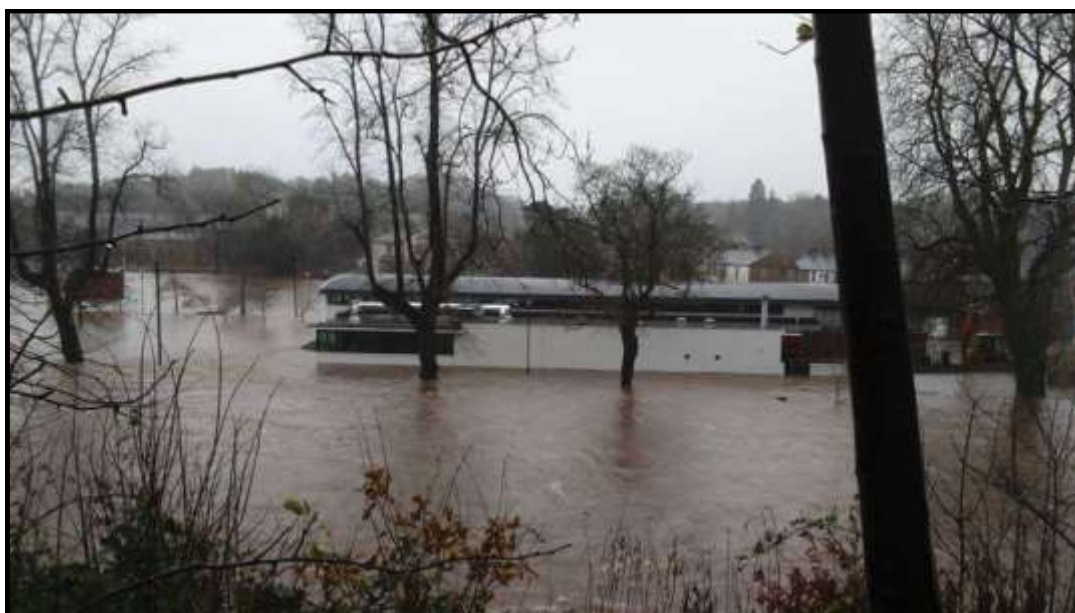
Photograph 21: River Eden at Appleby Leisure Centre
