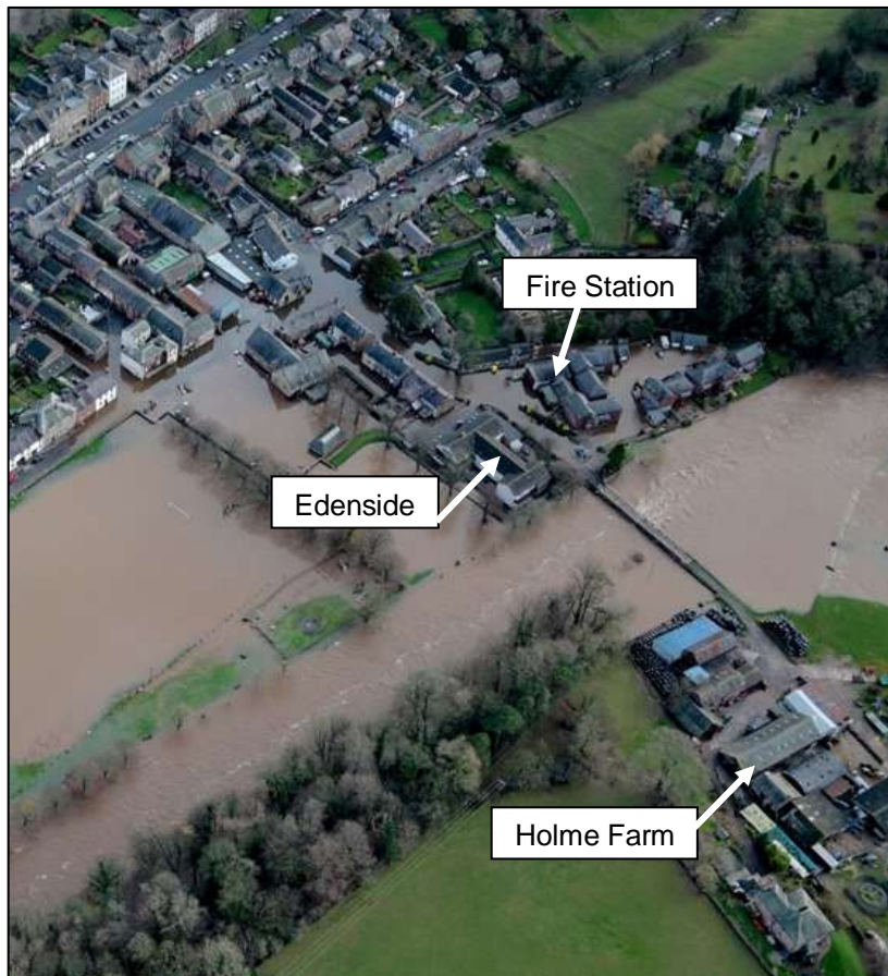
Photograph 7: Flood Extent on Holme Street
