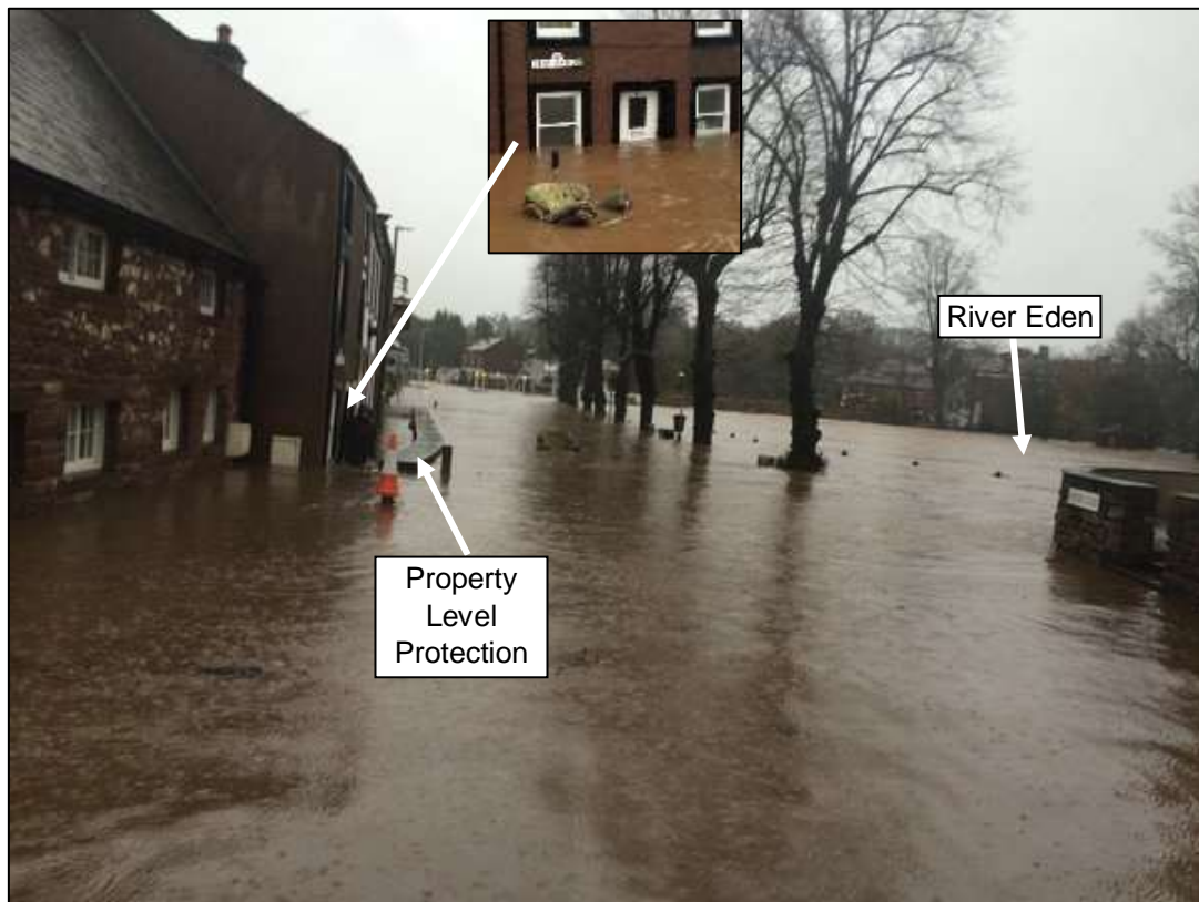
Photograph 3: Flooding at The Sands, Appleby
