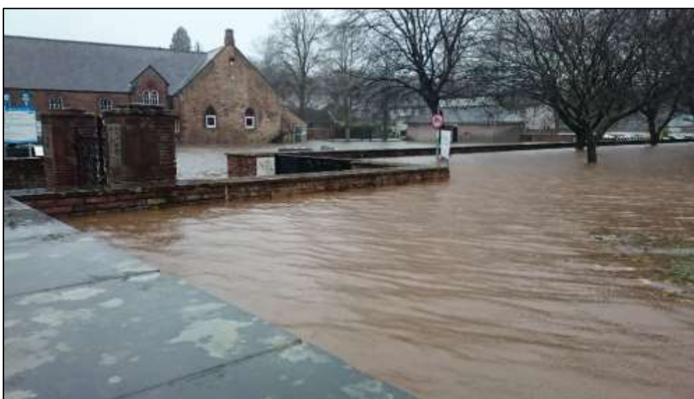
Photograph 29: Water ponding behind floodwall on Chapel Street
