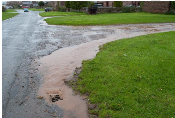
Photograph 16: Surface water discharging to highway gully outside Hollies
