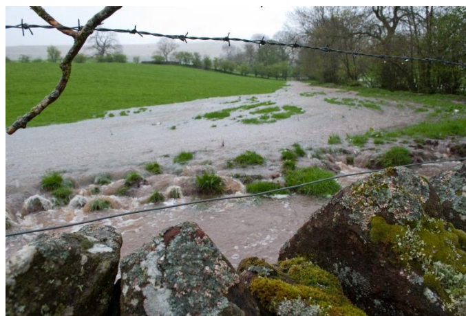
Photograph 9: Floodwater running across field above bridleyway
