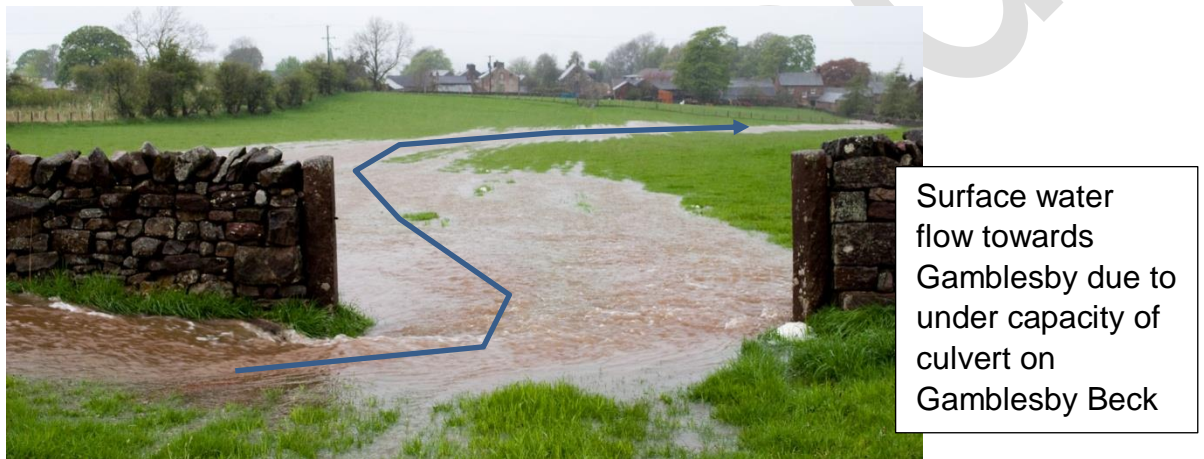
Photograph 5: Showing surface water flowing down field towards Gamblesby
