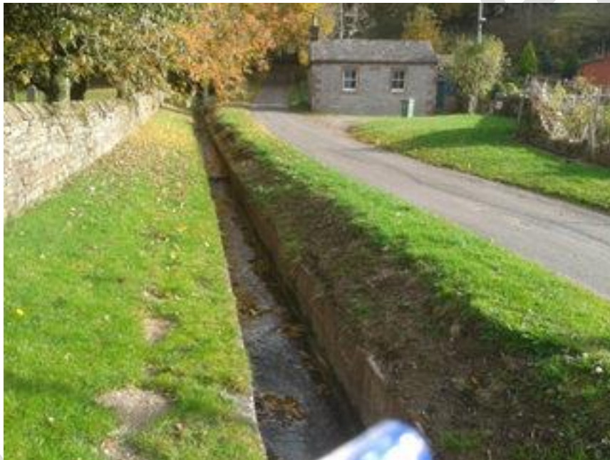
Photograph 4: Watercourse channel in normal circumstances parallel to Outhwaite Road
