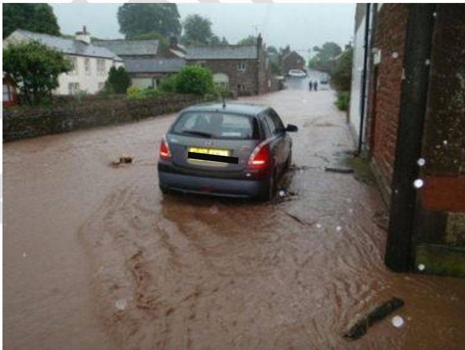
Photograph 7: Area where surface water collected causing flooding
