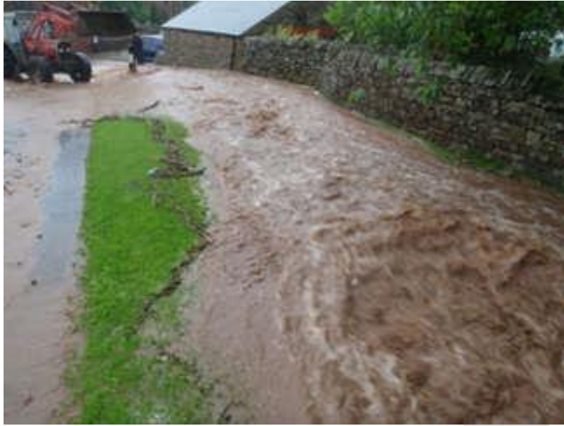
Photograph 3: Flow on 28 th June 2012 overwhelming culvert entrance
