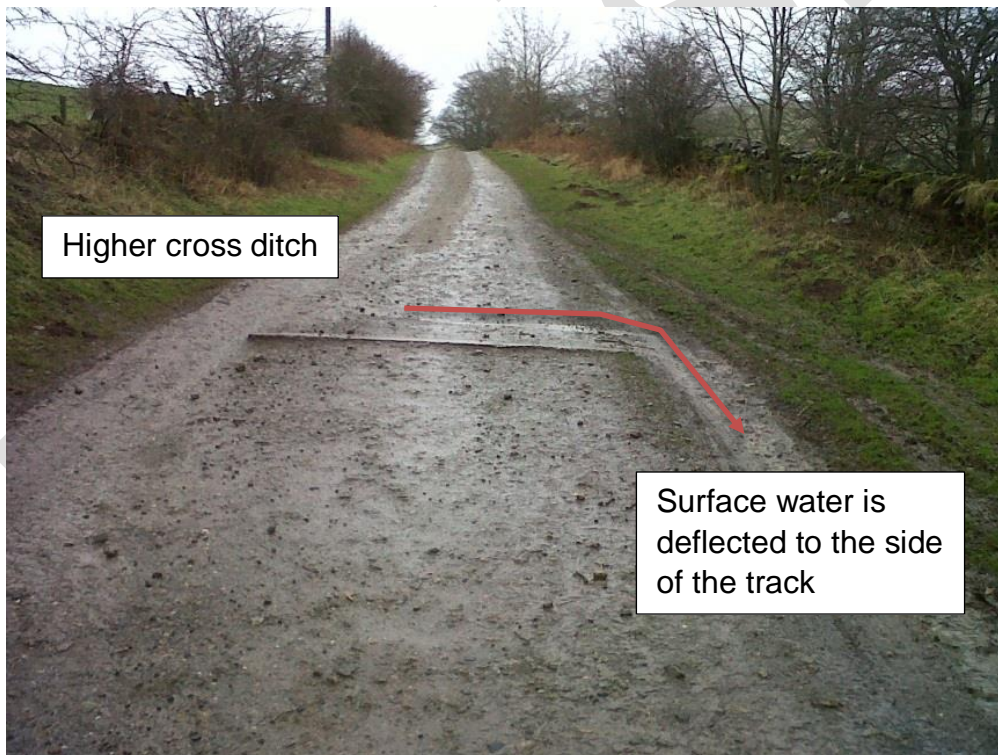
Photograph 3: Higher cross ditch deflects surface water to side of track
