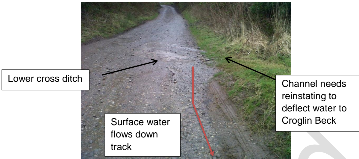
Photograph 4: Lower cross ditch
