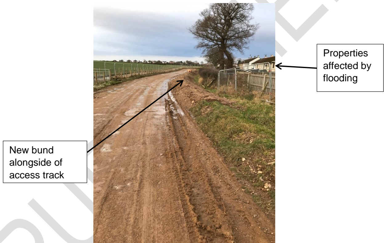
Photograph 6: Bund along new access track
