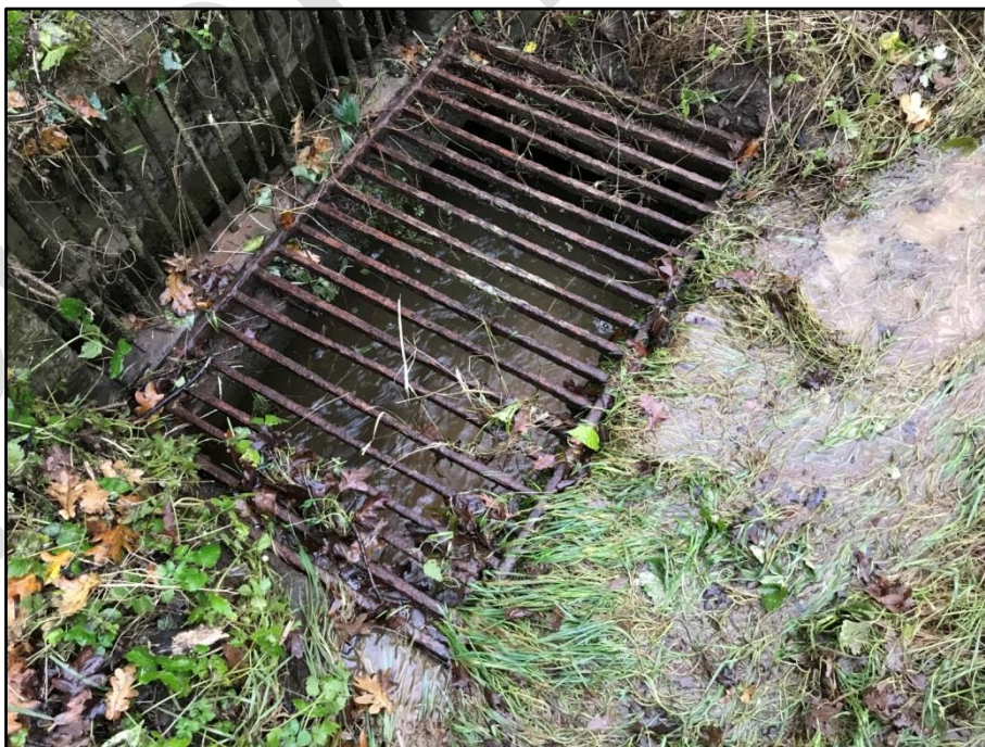
Photograph 4: Grid over culvert
