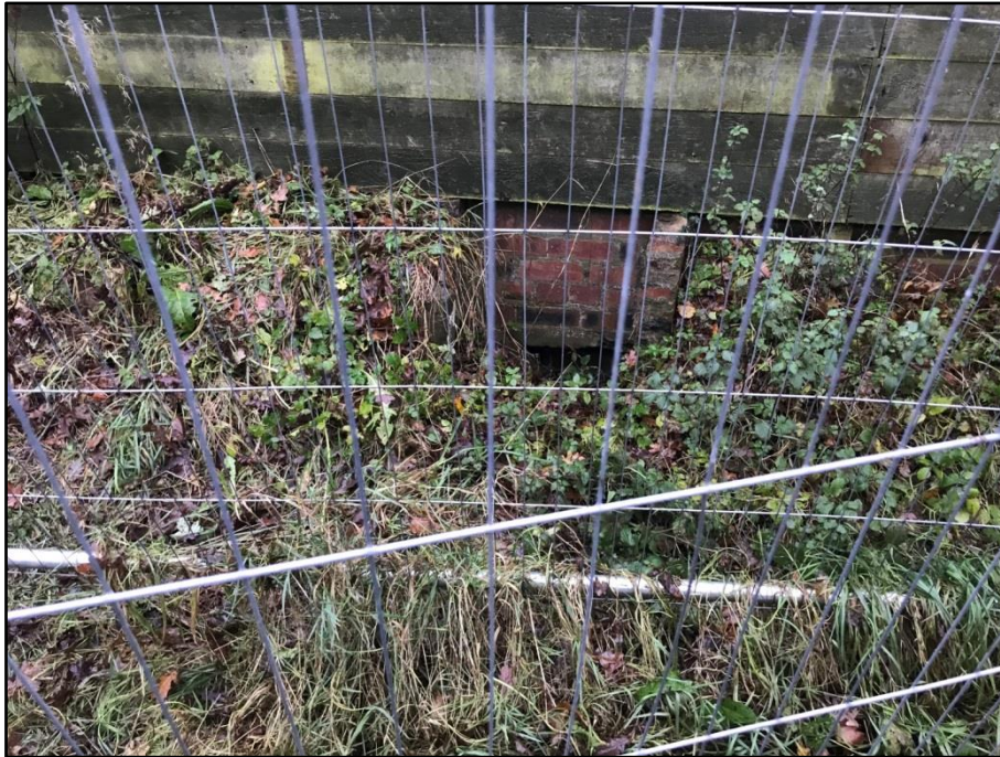
Photograph 3: Overflow drain to public sewer
