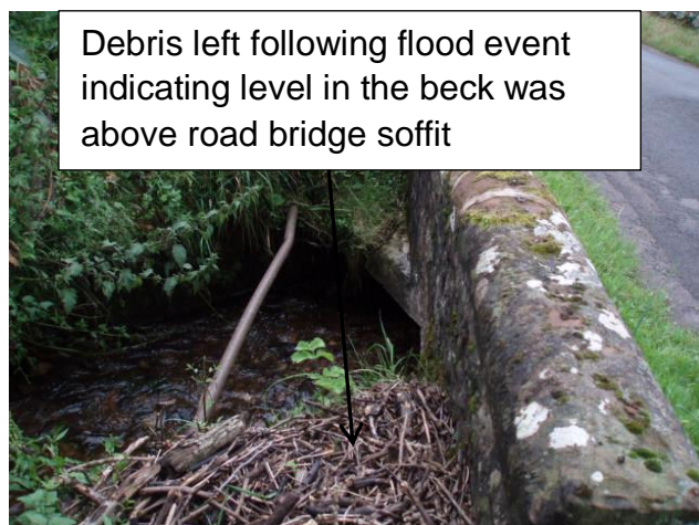
Photographs 6 & 7: Debris left next to the culvert near Rivendell and downstream culvert structure
