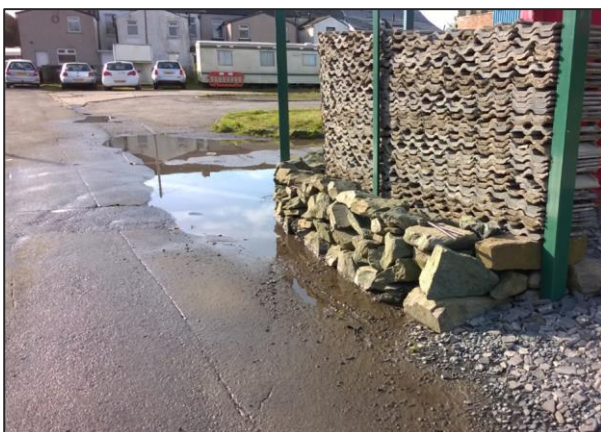
Photograph 11 (left): Standing water on collapsed chamber
