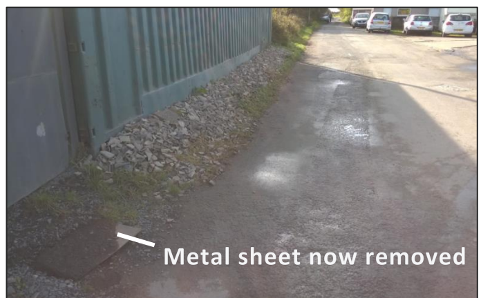
Photograph 11 (left): Standing water on collapsed chamber
