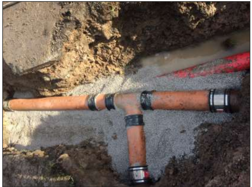
Figure 20: Highway drainage reinstated on Mainsgate Road. Photo courtesy of Electricity North West
