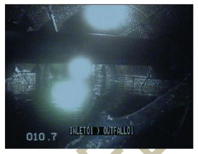
Figure 6. Picture from CCTV survey showing service pipe passing through the culvert and a branch caught on it
