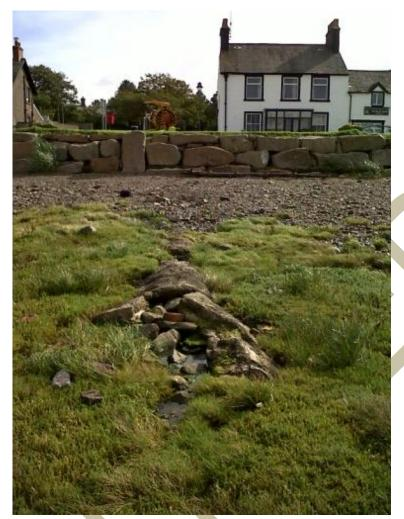
Figure 9. Broken pipe on beach carrying car park drainage (Outfall 2 in Figure 7).
