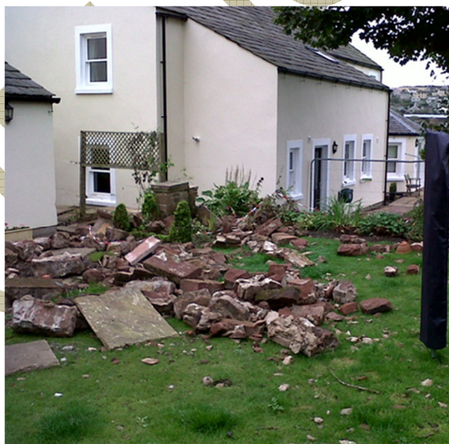
Figure 8. Devastation in the garden of Orchard House after the 30/8/12 flood knocked over walls
