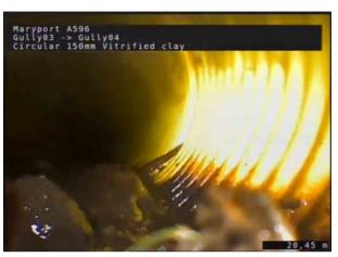
$2,\,00:03:07,\,20.16\;\text{m}$  Settled deposits, coarse, 30% cross-sectional area loss
