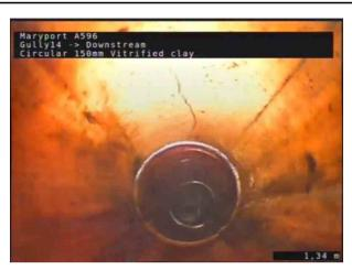
1, 00:00:19, 1.37 m Fracture, longitudinal at 12 o'clock
