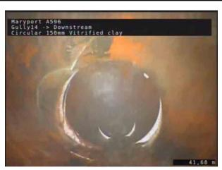
5, 00:04:40, 41.68 m Fracture, circumferential from 12 o'clock to 12 o'clock
