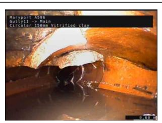
1, 00:00:11, 0.60 m Broken pipe from 9 o'clock to 3 o'clock
