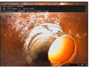
2, 00:01:20, 3.06 m Connection defective, position incorrect and intruding at 4 o'clock, 100mm dia, intrusion: 50%
