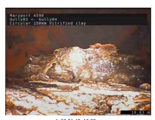
4, 00:01:45, 10.68 m Attached deposits, encrustation from 3 o'clock to 9 o'clock, 50% cross-sectional area loss, Grout
