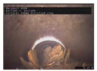
3, 00:01:22, 9.15 m Settled deposits, other, 75% cross-sectional area loss, Loose grout
