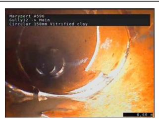
1, 00:00:14, 0.60 m Fractures, multiple from 12 o'clock to 12 o'clock
