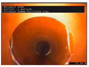
2, 00:01:54, 21.54 m Fracture, circumferential at joint from 2 o'clock to 4 o'clock
