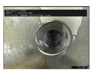
4, 00:01:54, 23.84 m Crack, longitudinal at 3 o'clock
