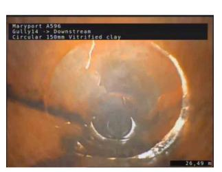
4, 00:03:32, 26.64 m Fractures, multiple from 12 o'clock to 12 o'clock
