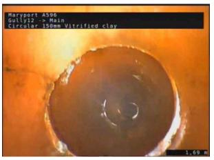
2, 00:00:28, 1.69 m Crack, longitudinal at 10 o'clock
