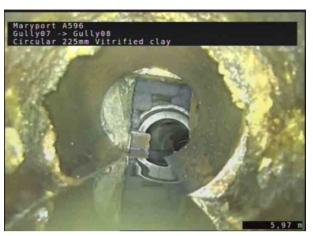
2, 00:00:47, 5.97 m Attached deposits, encrustation from 8 o'clock to 4 o'clock, 10% cross-sectional area loss
