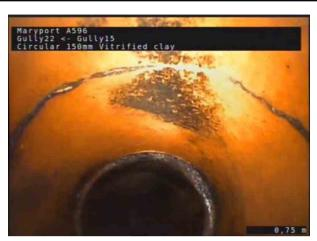
1, 00:00:14, 0.75 m Fracture, circumferential from 9 o'clock to 3 o'clock
