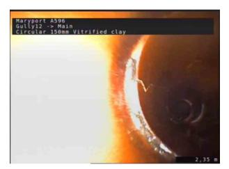
3, 00:00:33, 2.43 m Fracture, longitudinal at 10 o'clock
