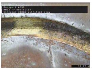
6, 00:02:49, 33.27 m Crack, longitudinal at 4 o'clock
