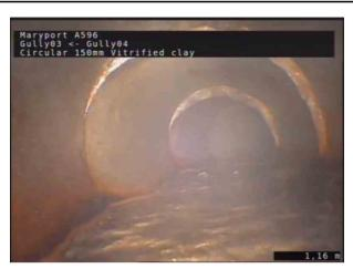
1, 00:00:33, 1.12 m Attached deposits, encrustation from 4 o'clock to 8 o'clock, 30% cross-sectional area loss, start
