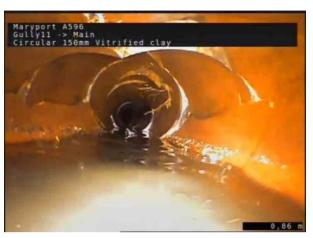
2, 00:00:18, 0.96 m Fractures, multiple from 12 o'clock to 12 o'clock
