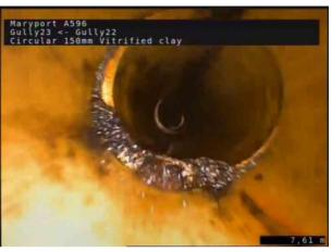
2, 00:01:21, 7.61 m Attached deposits, encrustation at joint from 5 o'clock to 9 o'clock, 15% cross-sectional area loss
