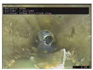
1, 00:00:40, 4.88 m Other obstacles, pipe material in invert from 4 o'clock to 7 o'clock, 10% cross-sectional area loss
