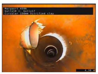
1, 00:00:33, 4.36 m Connection defective, connecting pipe is intruding at 10 o'clock, 100mm dia, intrusion: 20%
