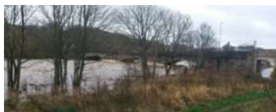
Figure 12- Workington Bridge during the flooding
