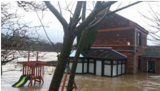
Figure 18 Flooding at Crossings House
