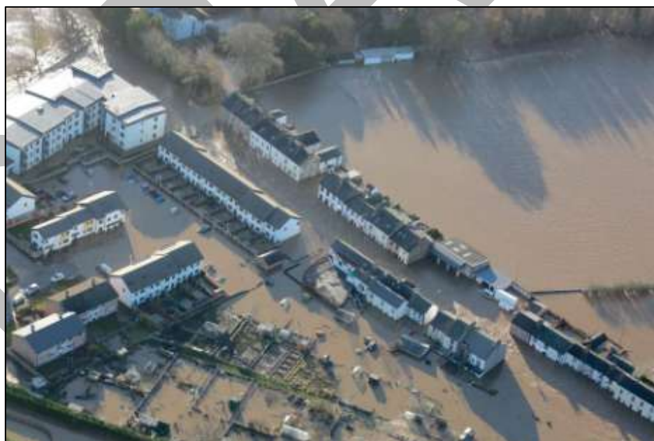
Figure 17-Gote Road area during event. Photograph provided by Peter Smith Photography. Taken 06/12/2015 12:35
