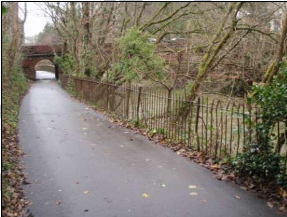
Figure 10-Riverbank between Victoria Jubilee Rail Bridge and Victoria Road Bridge (facing downstream). Taken 9/12/2015 at 11:40
