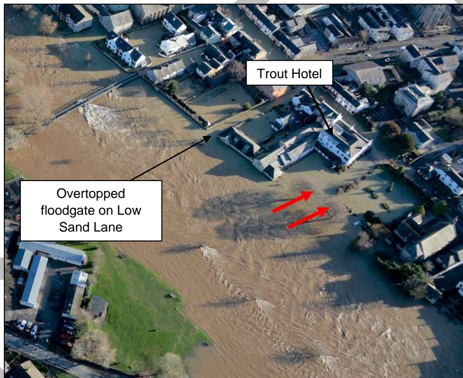
Figure 13-River Derwent at Main Street area highlighting flow route through the Trout Hotel car park. Photograph provided by Peter Smith Photography. Taken 06/12/2015 12:37
