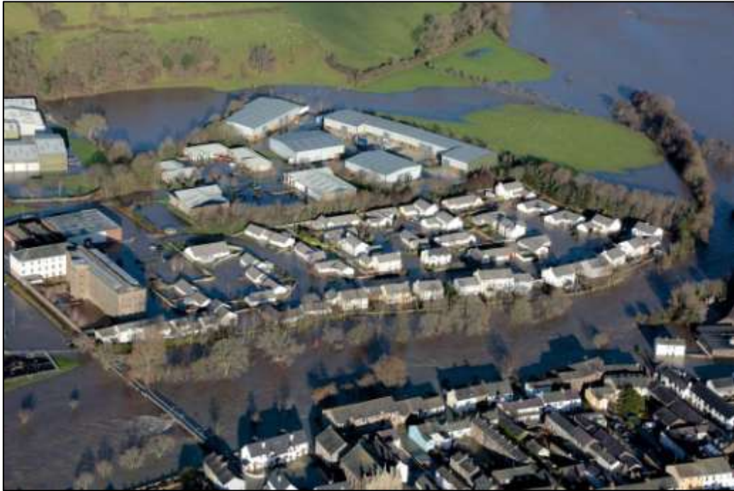
Figure 15-Derwentside Gardens during event showing flow route upstream of defence. Photograph provided by Peter Smith Photography. Taken 06/12/2015 12:37
