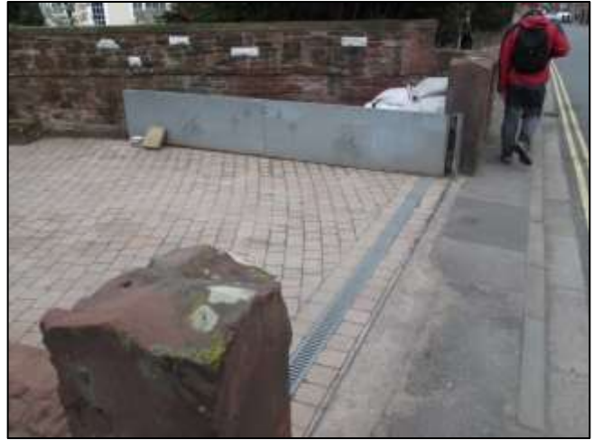
Photograph 8: Flood Gates on Station Road
