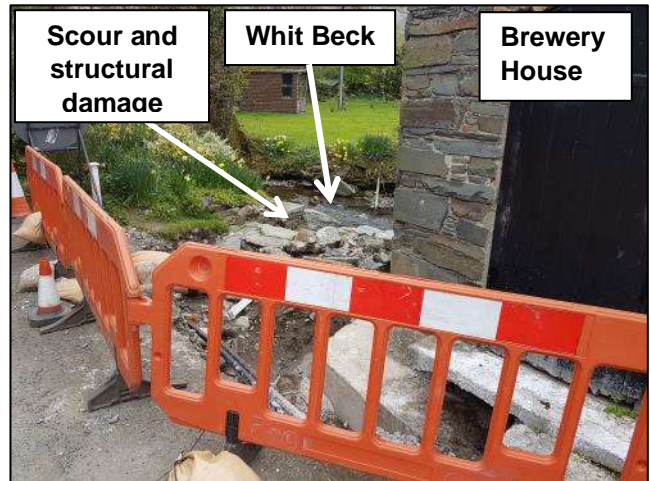
Photograph 12: Scour around properties on the westerly access road to the B5292
