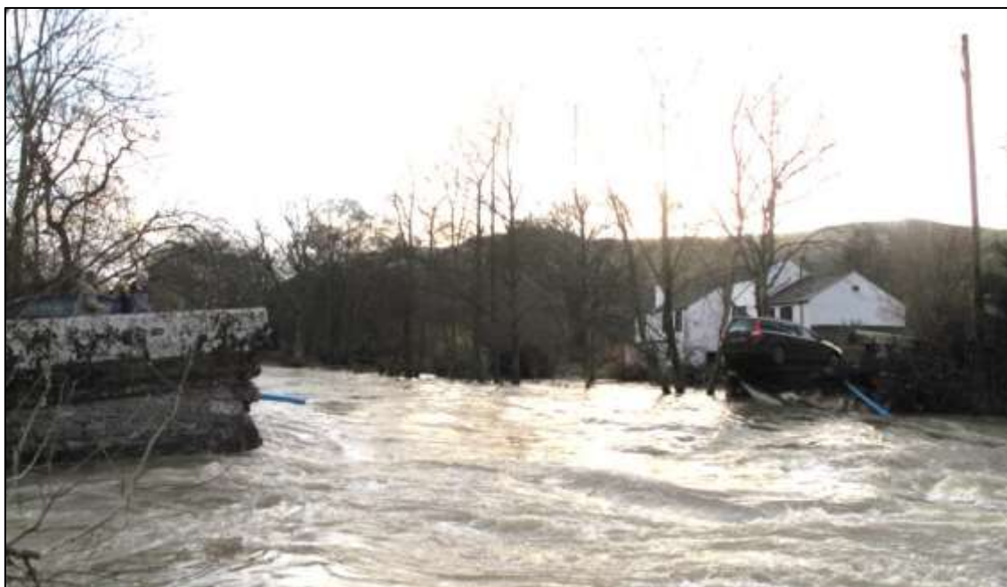
Photograph 4: Looking south towards the destroyed Lorton Bridge
