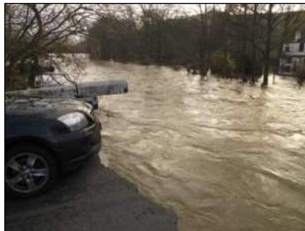
Photograph 3: Looking downstream from the destroyed Lorton Bridge
