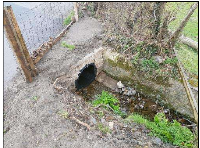
Photograph 20: Culverted ordinary watercourse
