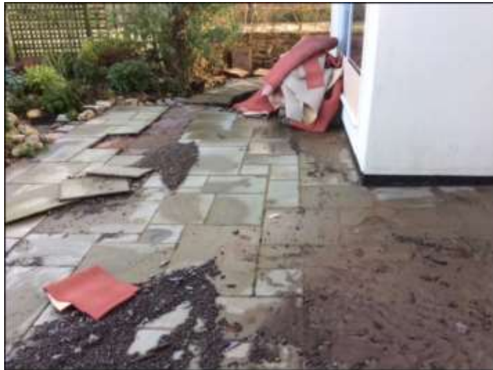
Photograph 9: Flood damage at Low Lorton
