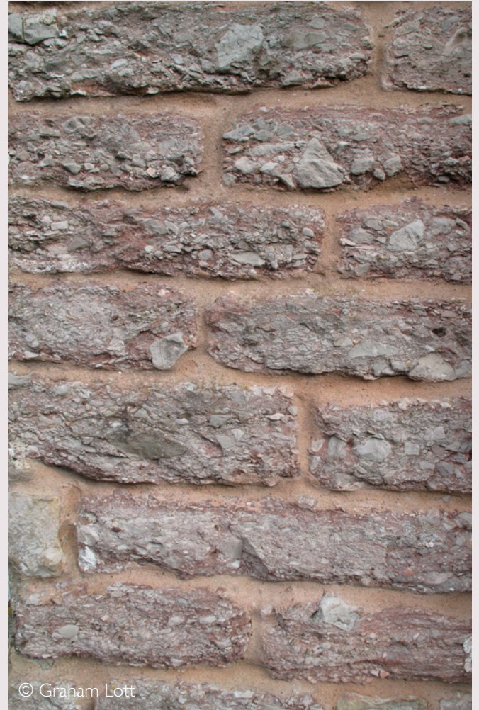
The highly distinctive ‘Brockram’ breccia, blocks of which are seen here in close-up, has been used to construct many of the buildings in the centre of Kirkby Stephen.
