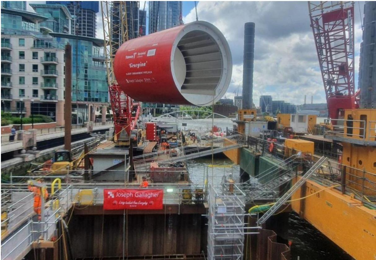
Figure 3 – tunnel shield being lifted into launch shaft
