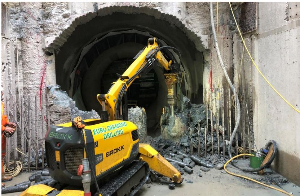
Figure 4: Brokk remote tunnel excavator
