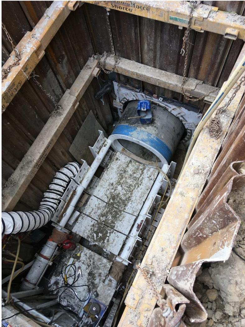
Figure 17 - similar arrangement of pipe jacking within pit bottom (note jacking spacers)
