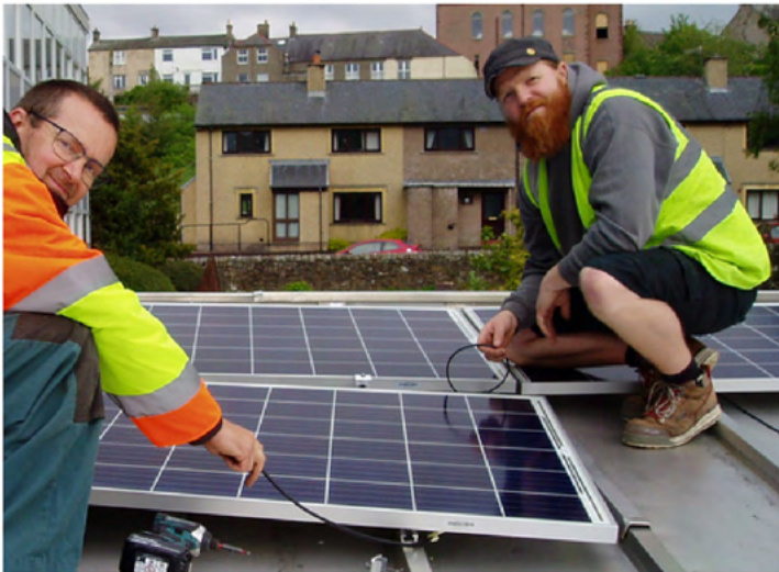
Installing solar panels
