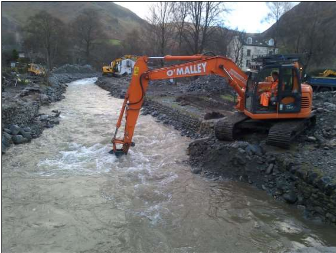
Figure 15-Gravel being removed from Glenridding Beck. Taken 10/12/2015 11:21
