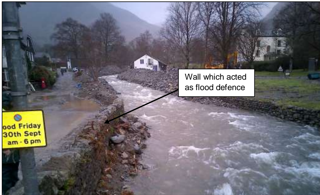
Figure 11-Wall along right bank of Glenridding Beck. Taken 9/12/2015 15:30
