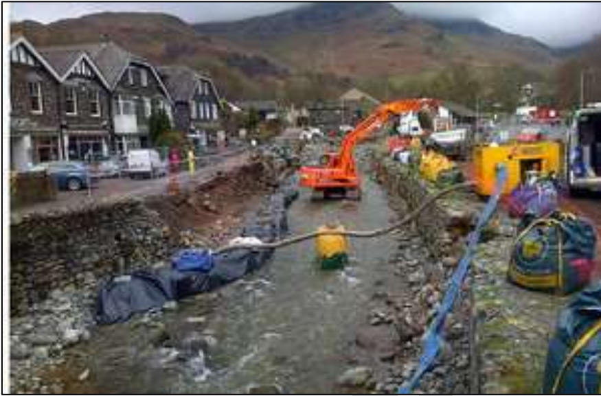
Figure 16-Construction underway of the new flood defence wall. Taken 14/12/2015
