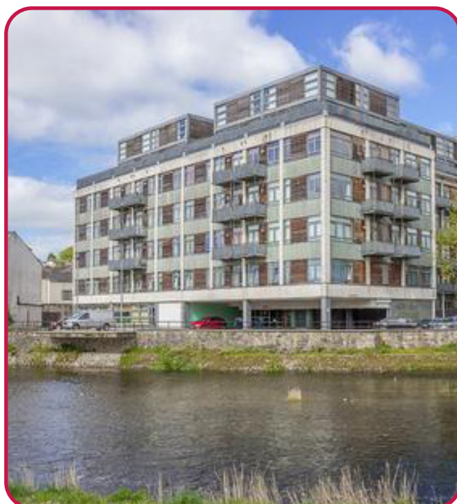
Sand Aire House, Kendal
