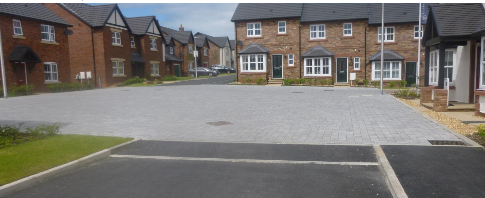
Figure SM1: A raised junction table within a new housing development
