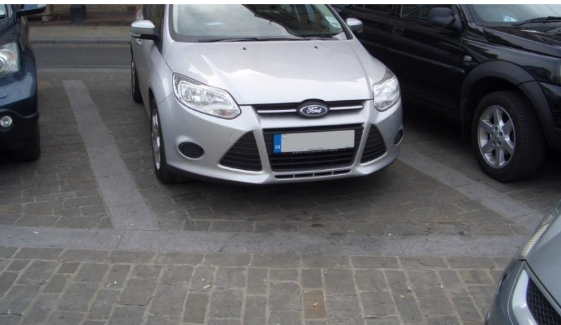
Figure P5: Parking bays marked out in quality materials
