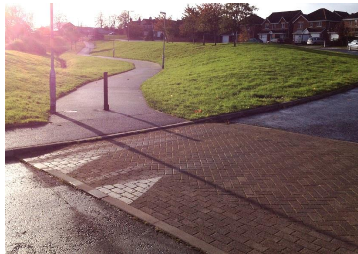
Figure SM3: Raised crossing helps cyclists and pedestrians across the carriageway, slows traffic on approaches and draws attention to the crossing point
