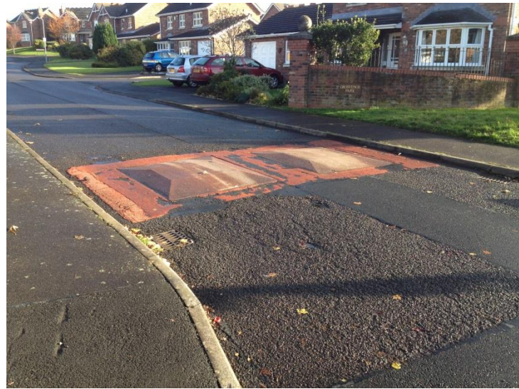
Figure SM2: Speed cushions applied retrospectively to a residential development diminish the road's character and impact negatively upon the place status of the road.
