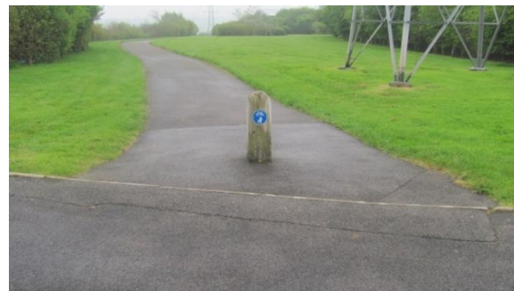
Concrete bollard with shared facility signage
