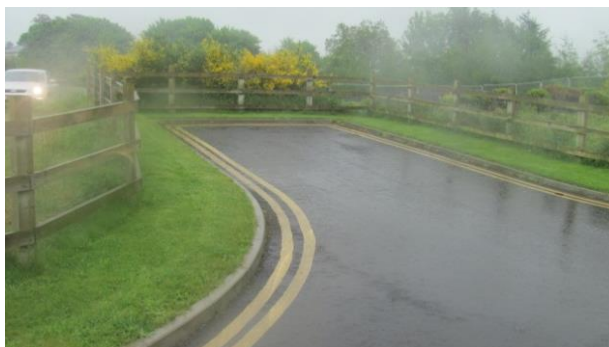
Turning facility treated with yellow line markings
