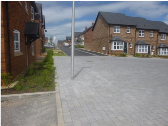
Figure L2: The position of the lighting column within a square puts it at risk of collision with vehicles and pedestrians
