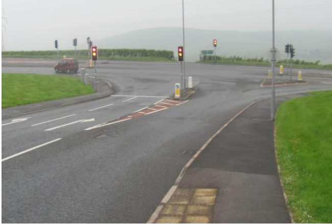
Signals at the entrance to West Lakes Science Park where it meets the A595
