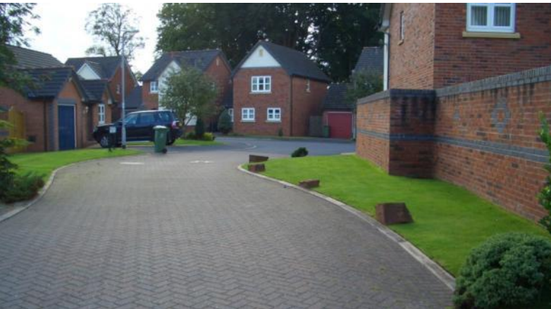
Figure P3: Retrospectively installed makeshift bollards
