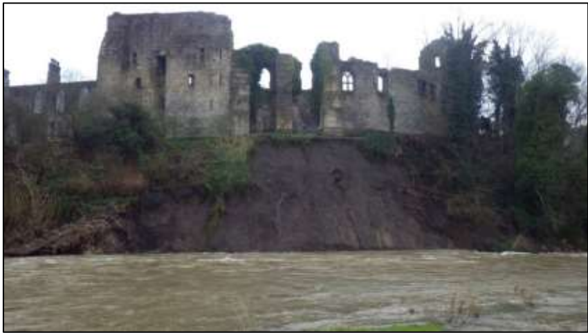
Photograph 1: Cockermouth Castle showing erosion to riverbank. Taken 21/12/2015
