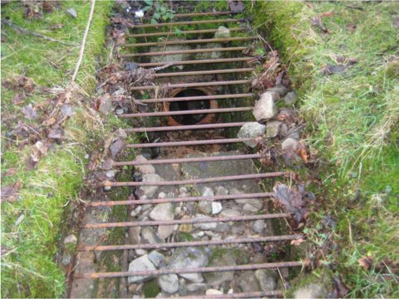
Figure 12 – Culvert inlet and trash screen upstream of Pedro's
