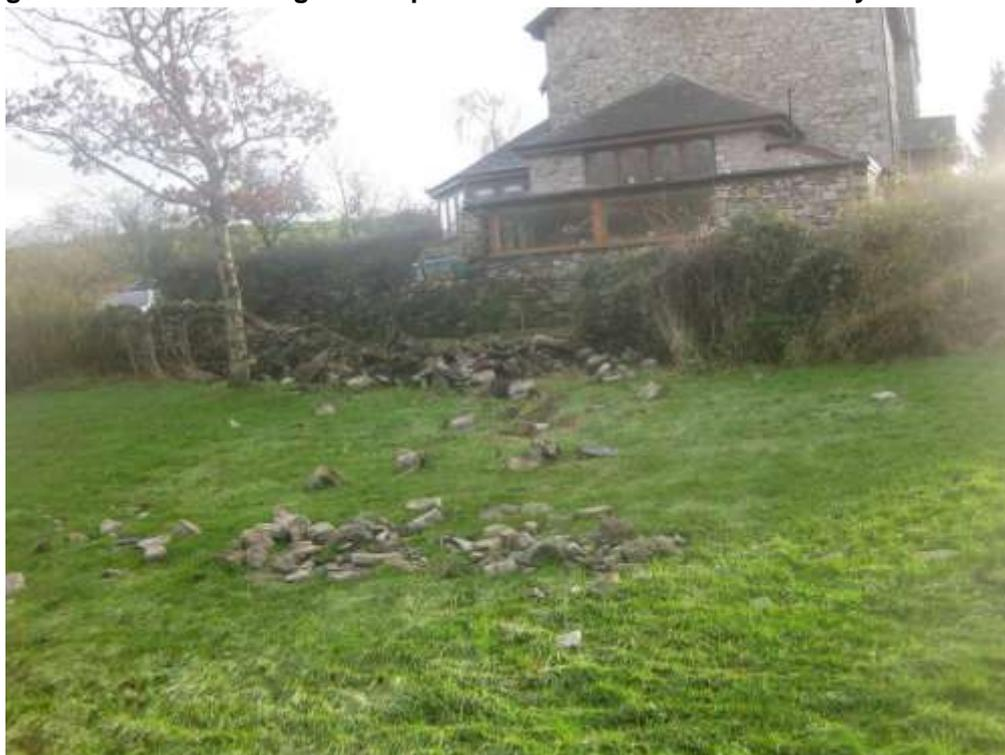
**Figure 16 – Demolished dry stone wall opposite Stainton Lodge, showing the flow route from the highway to Stainton Beck**
