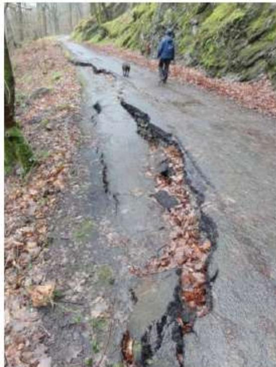
**Figure 10: The top of the Brundholme Woods landslide visible in the minor road through the woods.**
