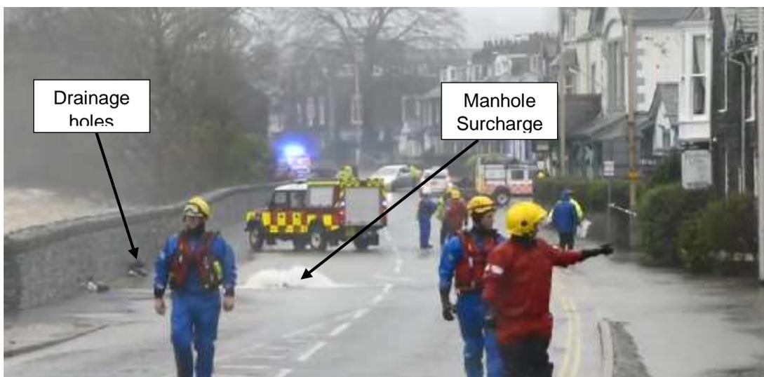
**Photograph 12: Manhole surcharge and flooding through drainage holes at the base of the flood defence wall on Penrith Road**
