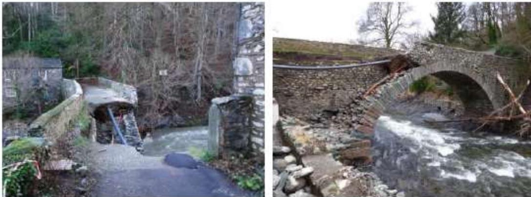
**Figure 12: Damage to bridge in The Forge area.**
