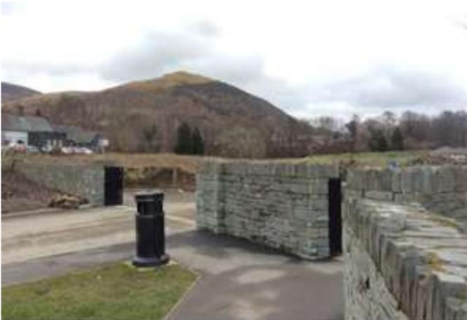
**Photograph 30: Crosthwaite Road flood defence wall**
