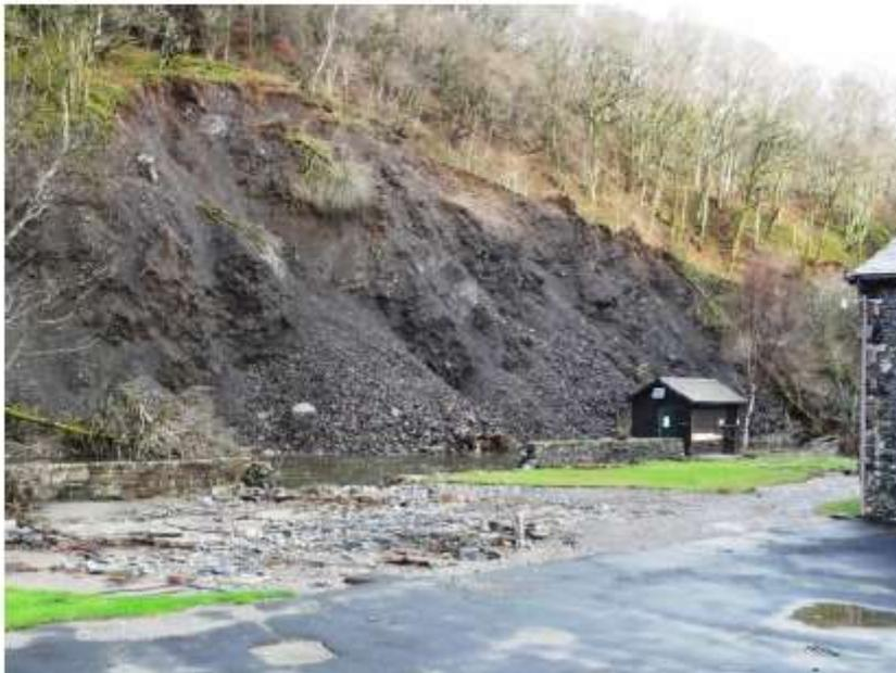
**Figure 11: Part of the bottom of the Brundholme woods slope where the river has eroded the bottom of the slope (the brown hut is the EA gauging station).**
