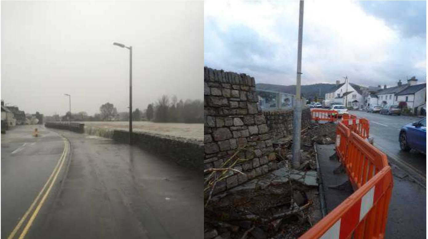
**Photograph 25 and 26: Flooding at High Hill Road - Floodwall first overtopped where glass panels finish (left) and scoured footpath (right)**
