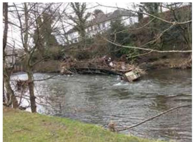
**Photographs 18 and 19: Riverside view of Youth Hostel (left) and washed out footbridge resting on left bank abutment (right)**
