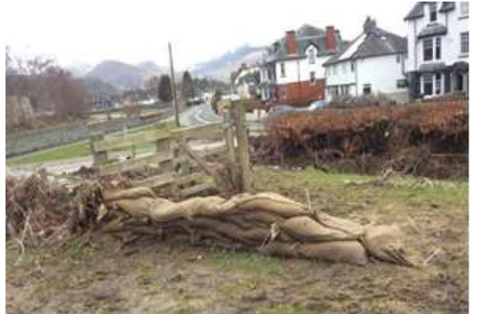
**Photograph 31: Crosthwaite Road flood defence embankment that was overtopped**
