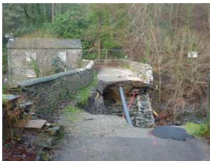
**Photograph 6: Forge Bridge Partially Collapsed**
