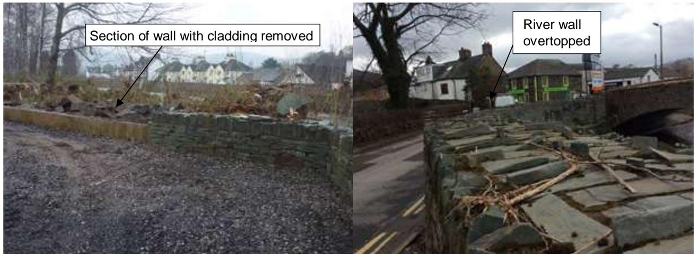
**Photographs 20 and 21: River overtopped its bank/flood wall at Southey Hill Estate (left) and the river wall overtopped at upstream of Greta Bridge (right)**
