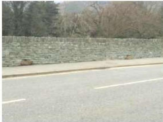
**Figure 22: Drain holes left under flood defence wall (sandbags in place).**
