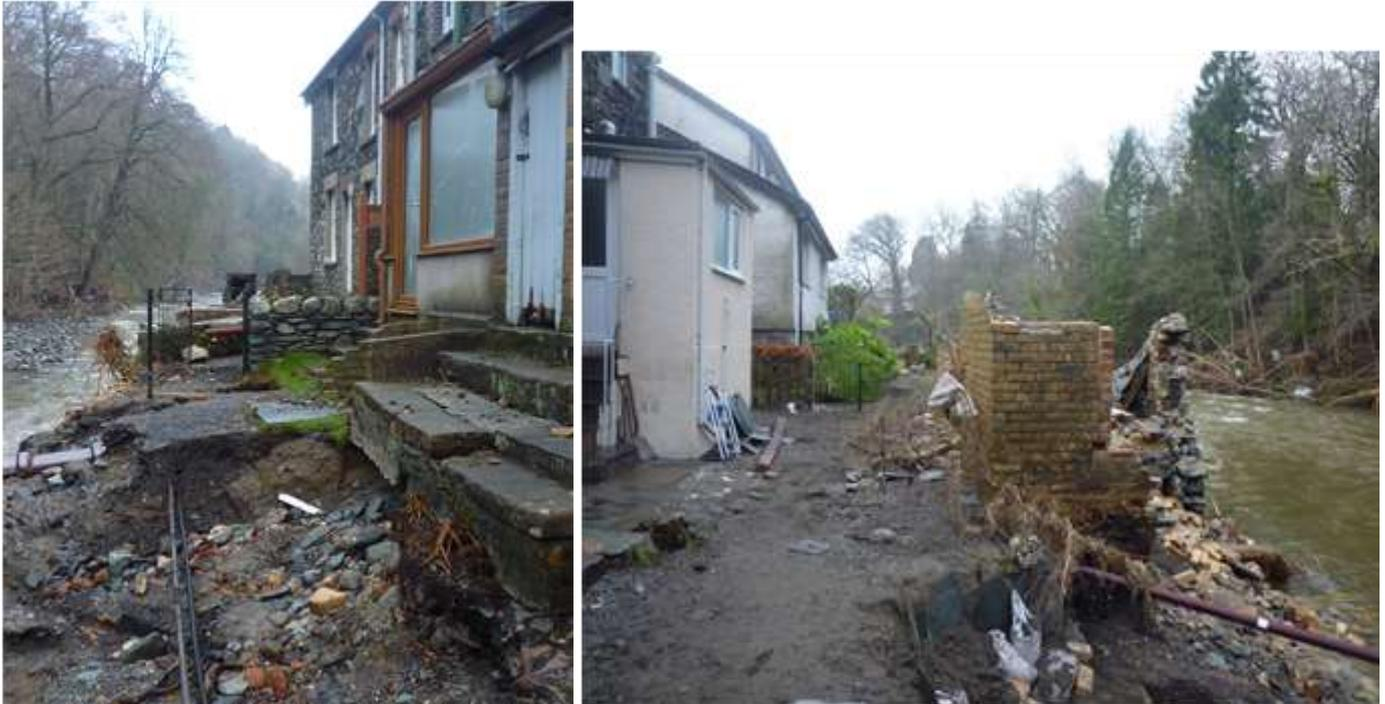
**Photographs 7 and 8: Scour damage to the rear of properties**
