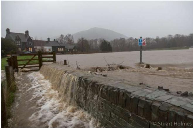
**Photograph 32: Overtopping of flood defences on Crosthwaite Road**
