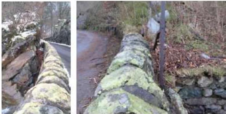
**Figure 6: Photographs of flood debris close to the top of the wall that runs along the top of the dam at Thirlmere.**
