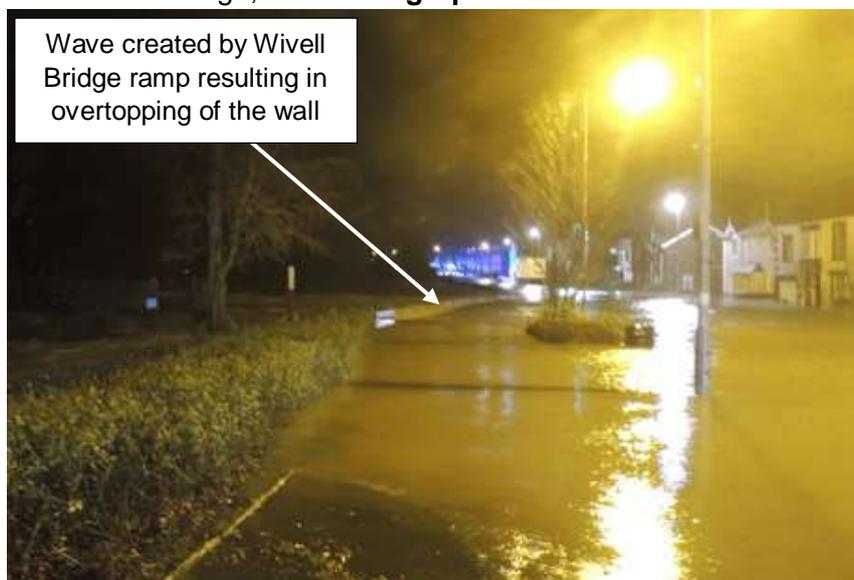
**Photograph 13: Wave created by the access ramp on the left bank at Wivell Bridge**
