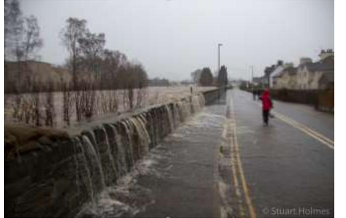
**Photograph 33: Overtopping of flood defences on Crosthwaite Road**
