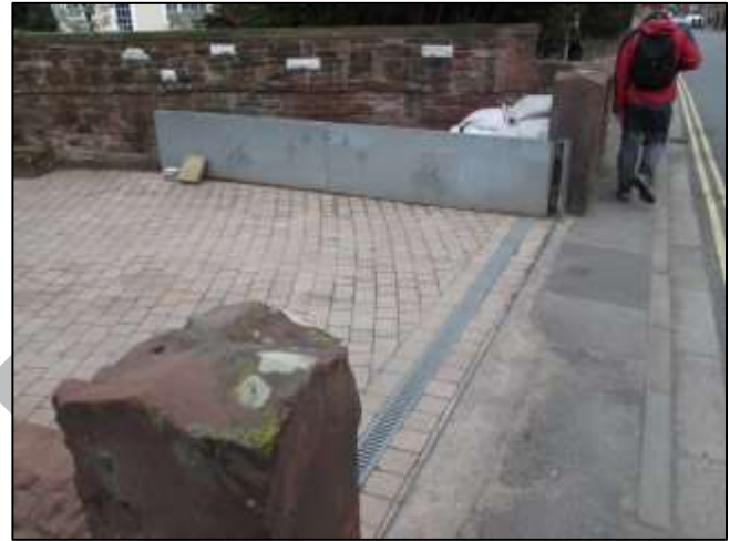
Photograph 8: Flood Gates on Station Road
