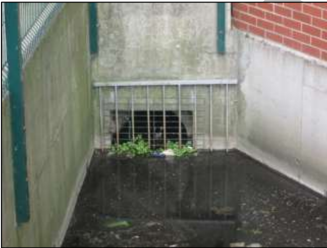
Photograph 14: Lidl Trash Screen
